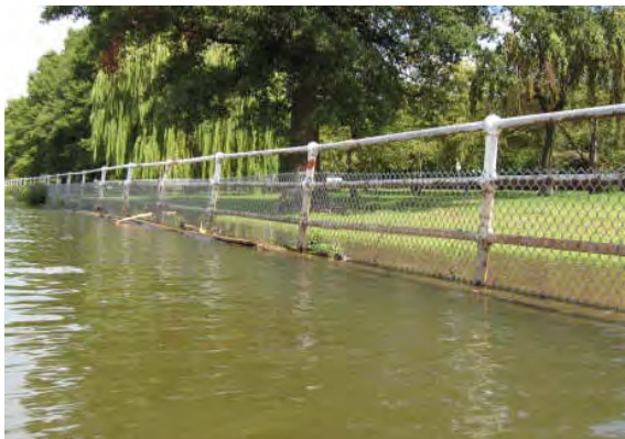
The Potomac Park seawall is sinking and needs repairs.
