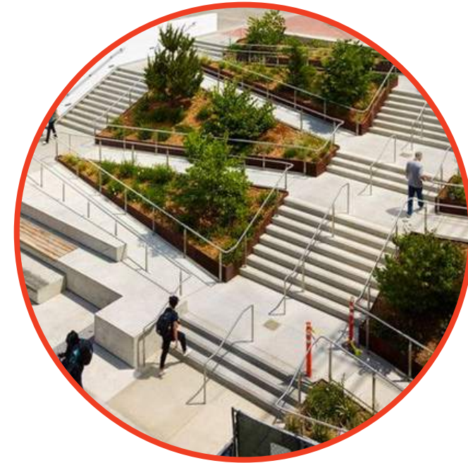
CONCRETE RAMPS WITH HANDRAILS
