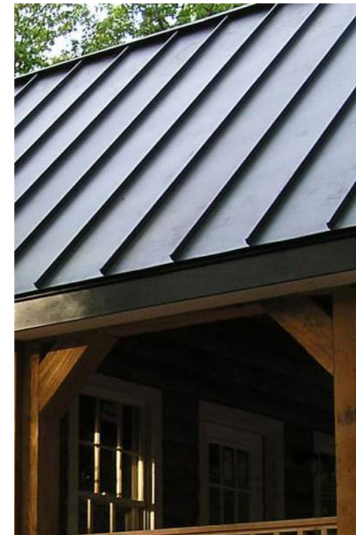
STANDING SEAM ROOF
