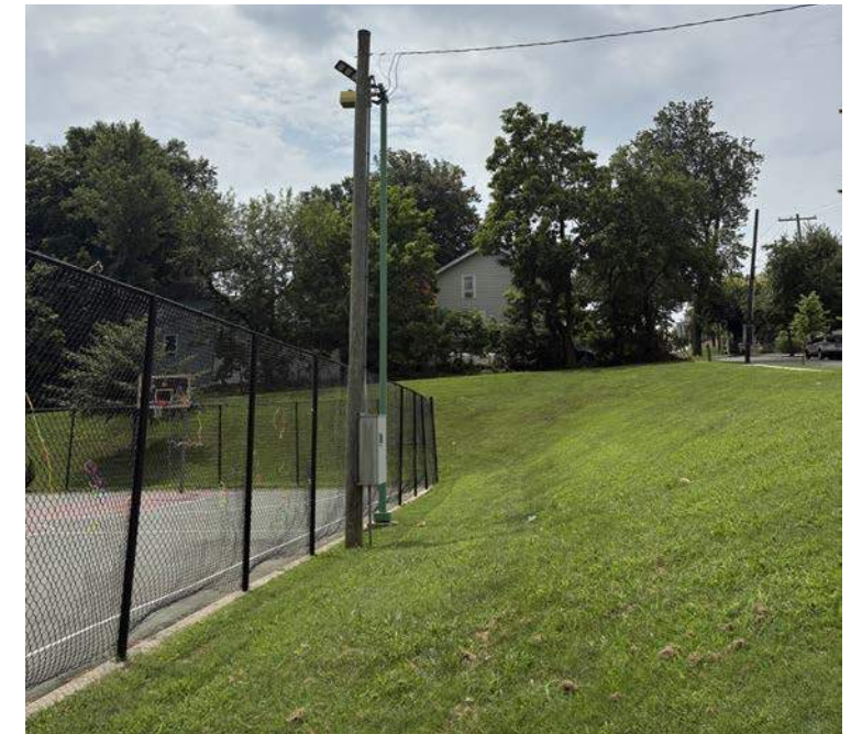
2. SLOPE AT 20TH ST
