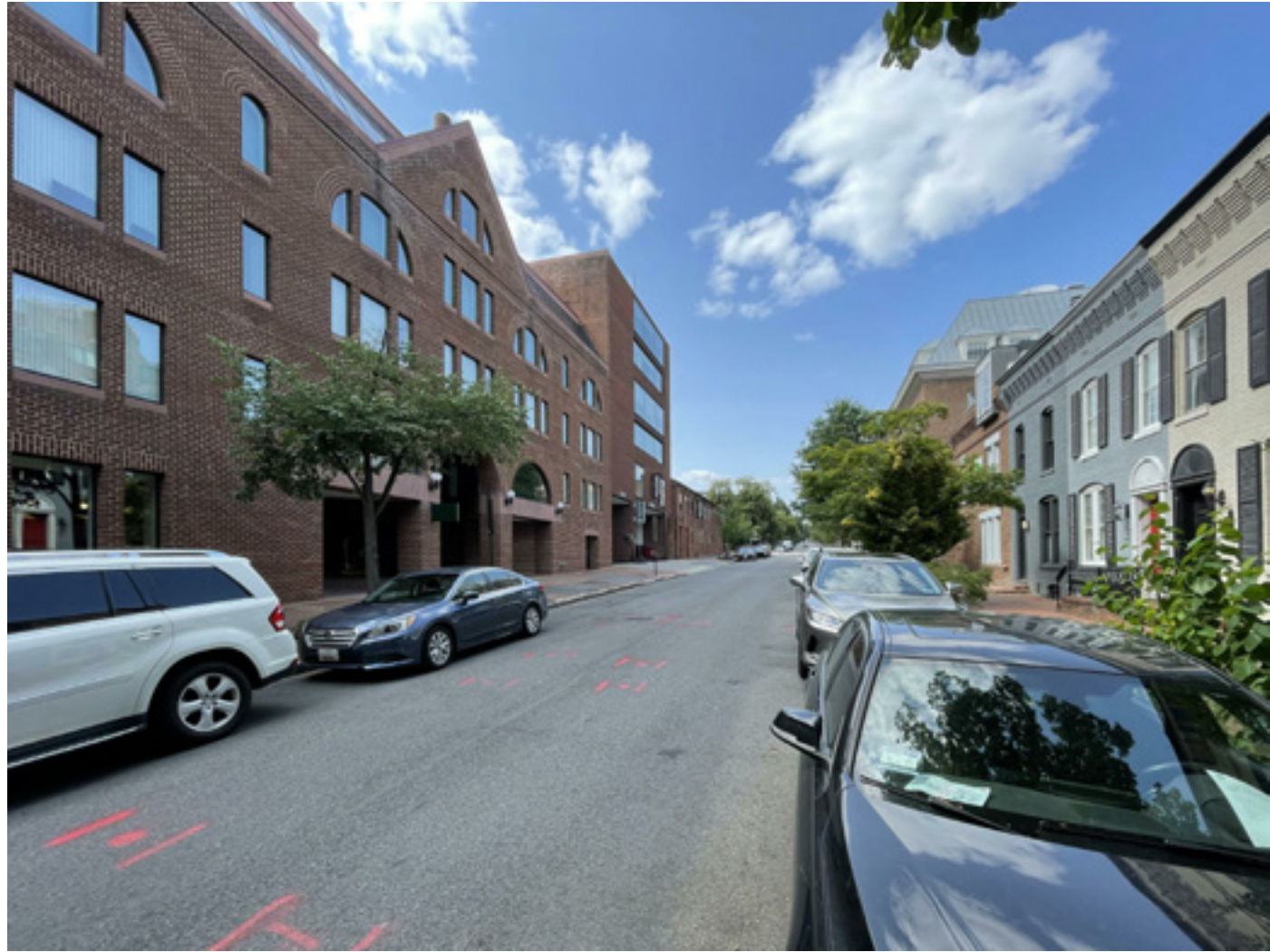
EXISTING - 30TH ST. LOOKING NORTH 2 BLOCKS AWAY
