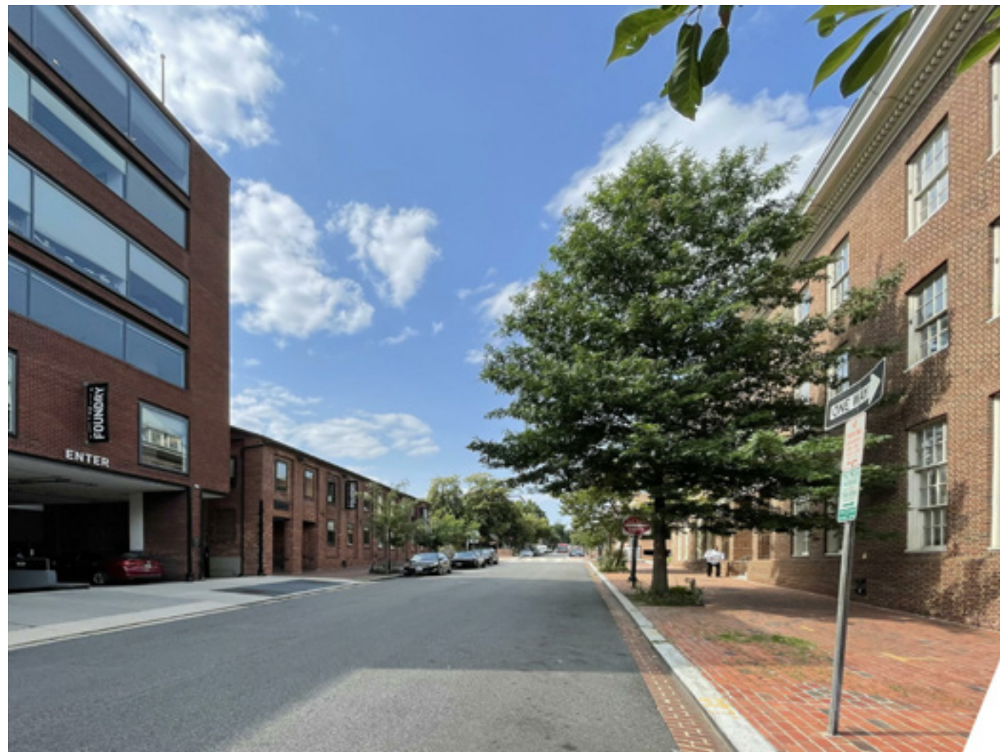
EXISTING - 30TH ST. LOOKING NORTH 1 BLOCK AWAY
