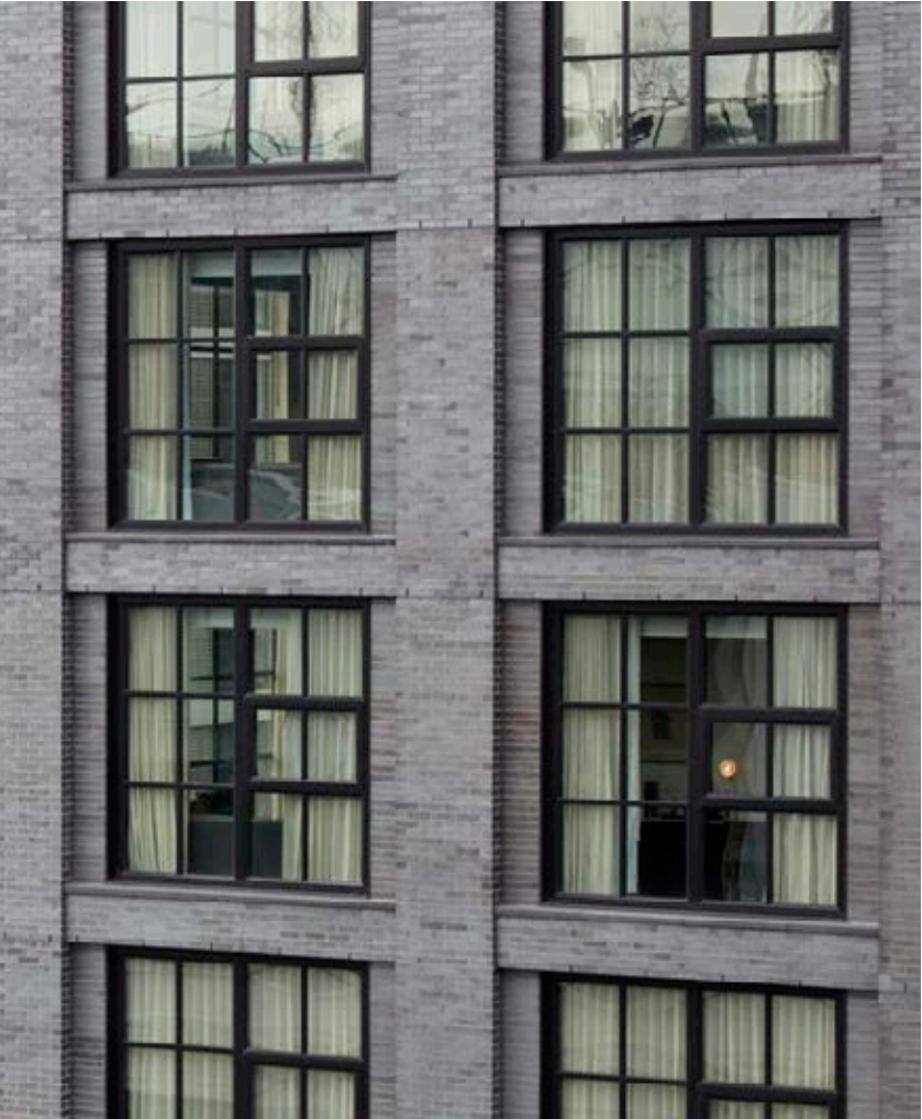
INSTALLED PRECEDENT WINDOW SYSTEM PHOTO
