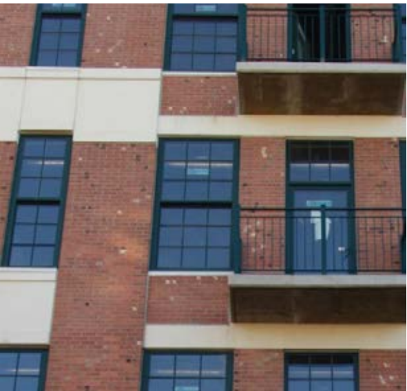
INSTALLED PRECEDENT WINDOW SYSTEM PHOTOS
