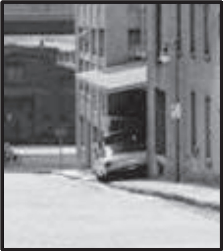
HISTORIC BUILDING ENTRY ELEMENT
