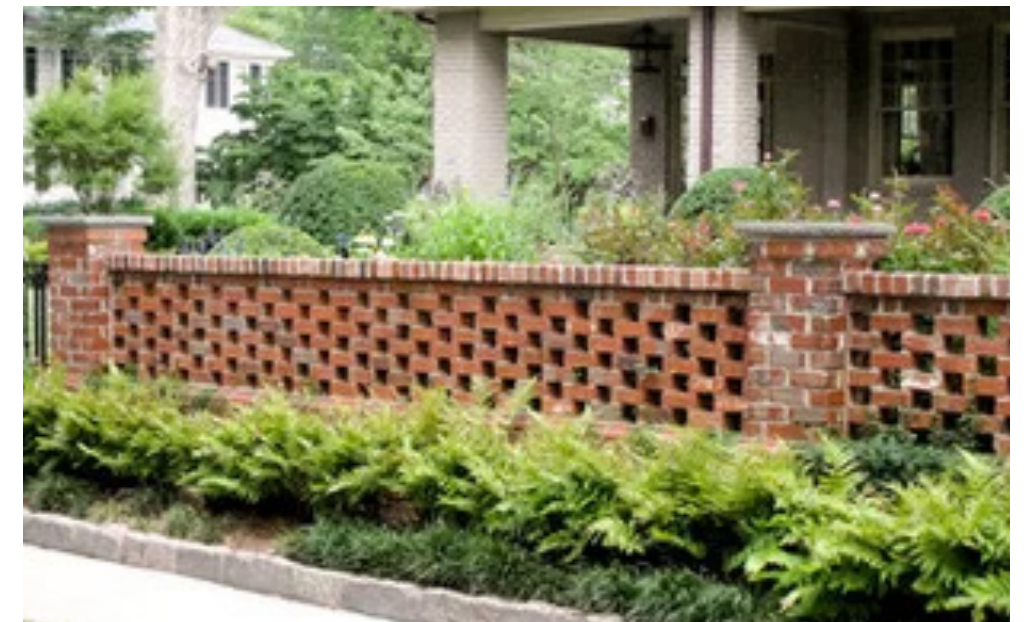
Perforated brick walls delineate and buffer spaces
