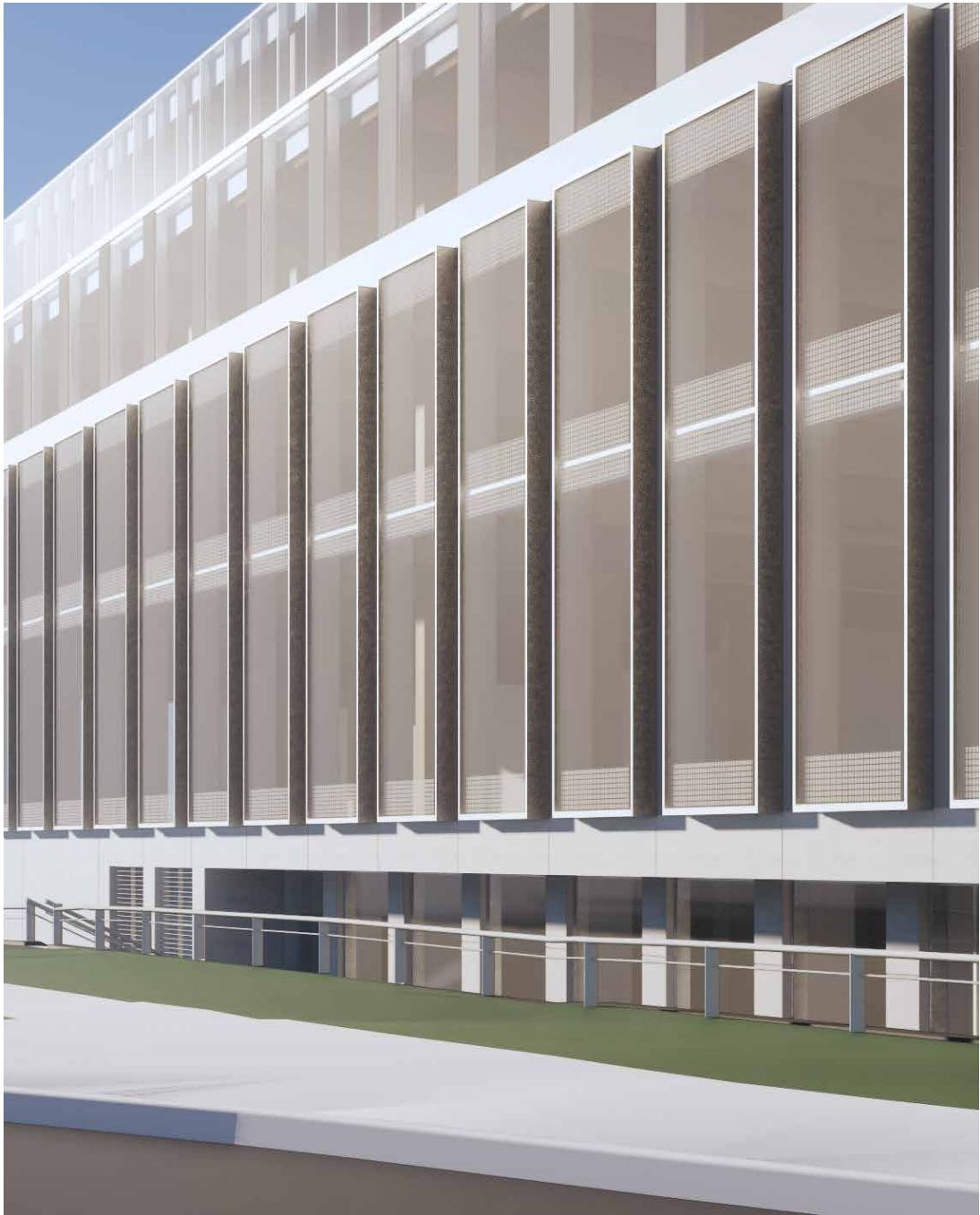
FRB-East Addition bays project 14" from the face of adjacent glazing panels
