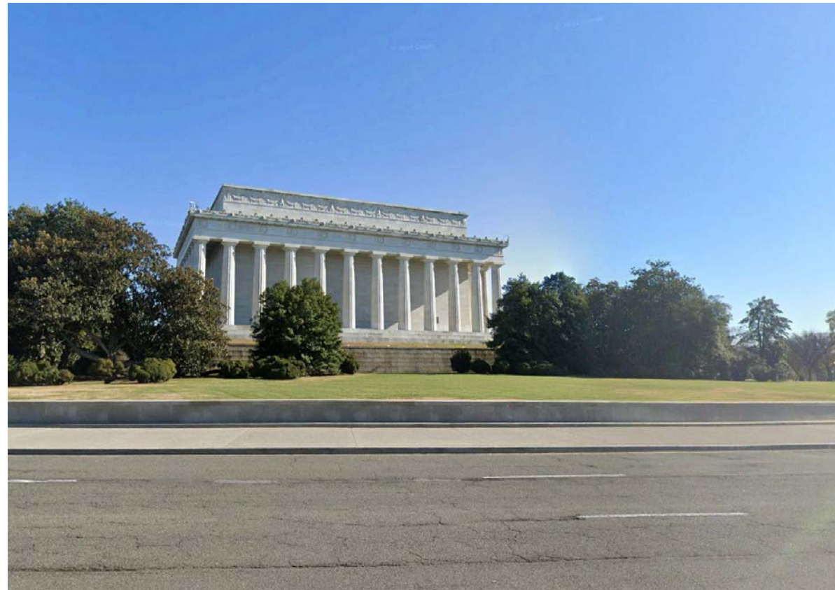
Images show the Lincoln Memorial site security methods from multiple angles. Security interventions include site walls and bollards.
