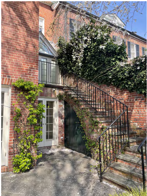
A1 3 EXISTING SIDE VIEW OF STAIRS
