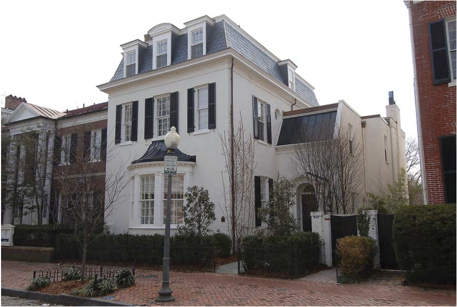
A2 2 EXISTING SIDE VIEW OF SIDE ELEVATION
