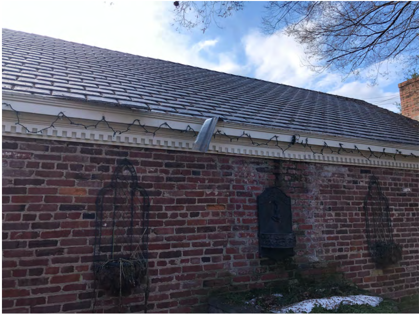
B2 2 EXISTING VIEW OF FOUNTAIN
