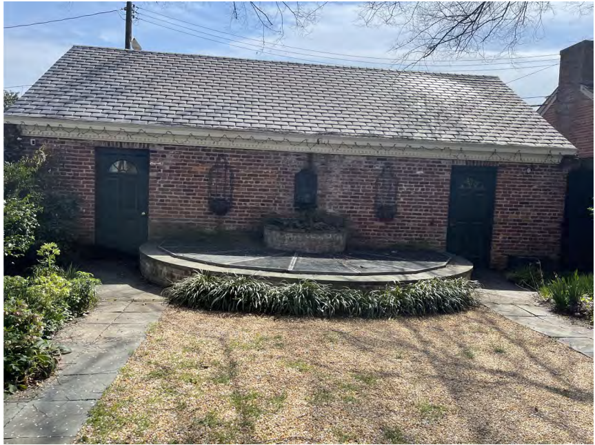
B1 2 EXISTING VIEW OF GARAGE AND FOUNTAIN
