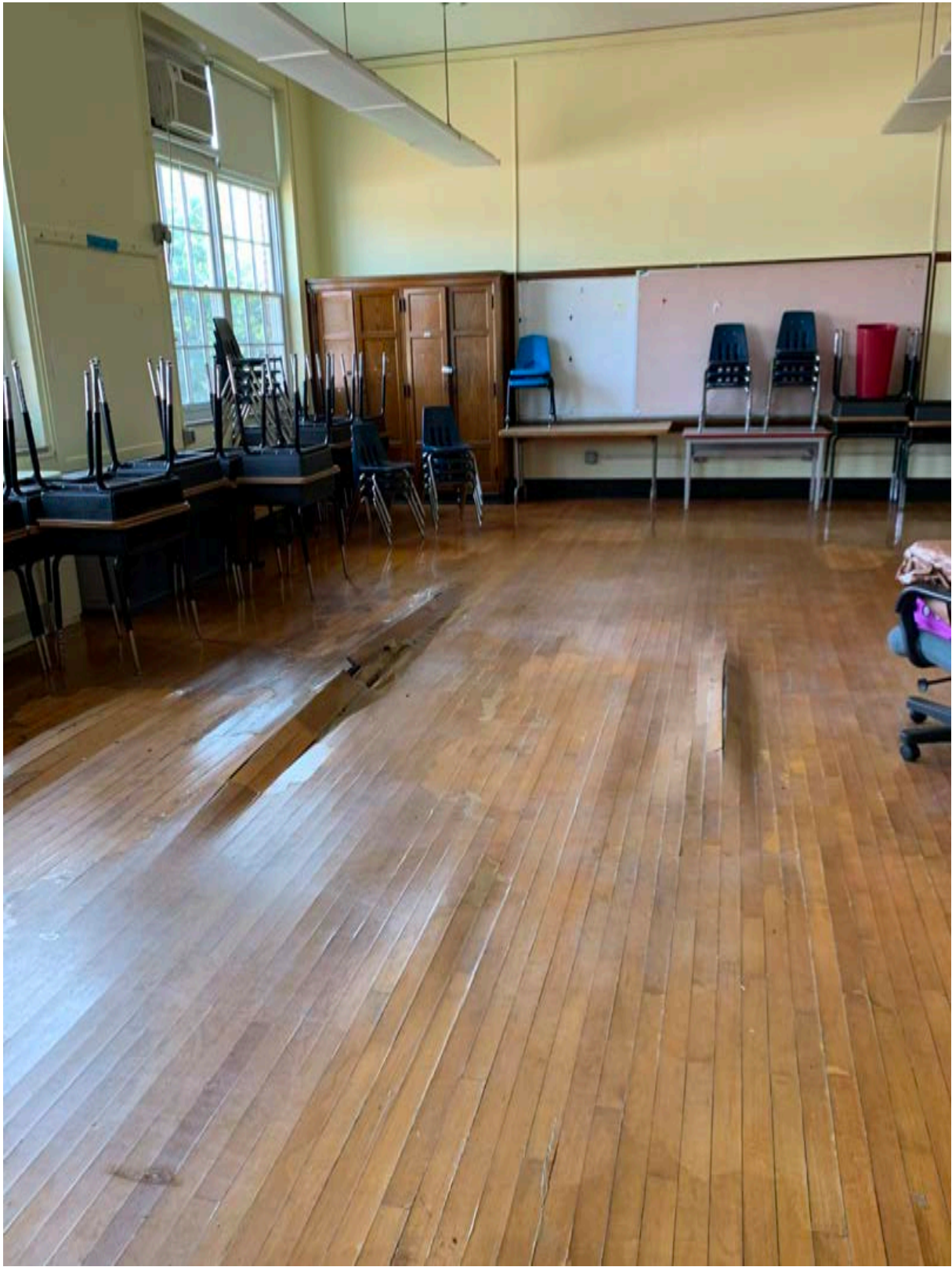
WARPED WOOD FLOORING IN CLASSROOM
