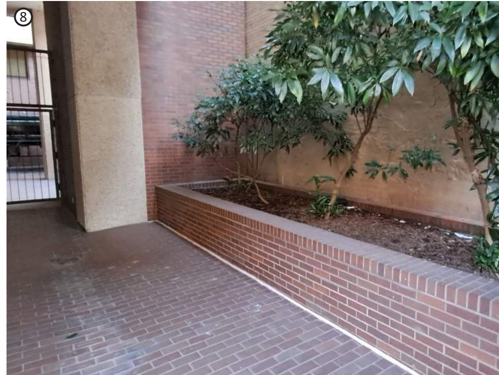
8 MARGINAL HIDDEN SPACES CAN BE FOUND IN THE WESTERN PART OF THE BUILDING
