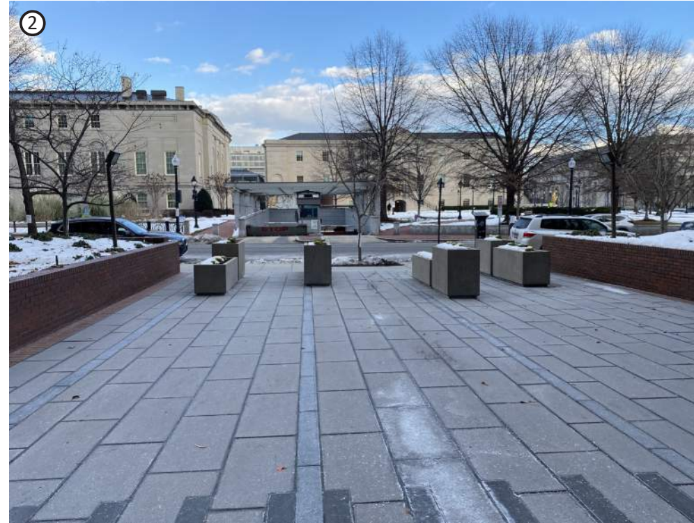
② CONCRETE PLANTERS AT THE MAIN ENTRANCE PREVENT HIGH FOOT TRAFFIC AND VEHICLES FROM ENTERING. SPECIAL PAVING IS SHOWN
