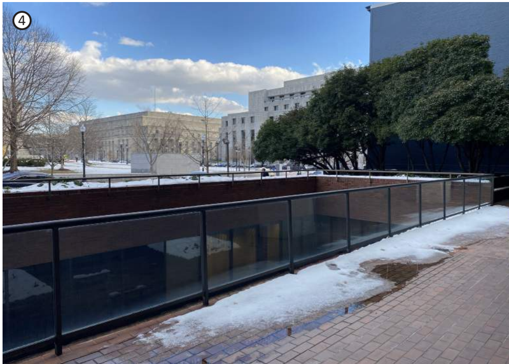
④ CELLAR COURTYARDS ARE SURROUNDED BY UNSTURDY GLASS AND METAL RAILINGS
