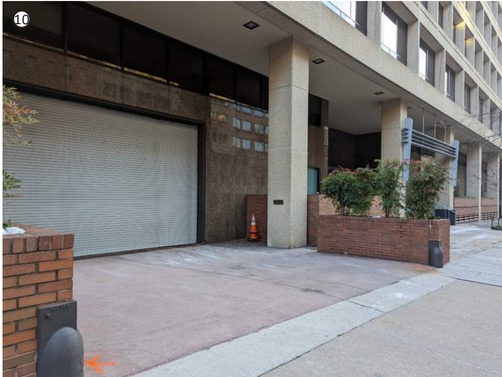
10 THE BACKSIDE OF THE BUILDING IS RESERVED FOR LOADING AND ACCESS TO THE PARKING GARAGE
