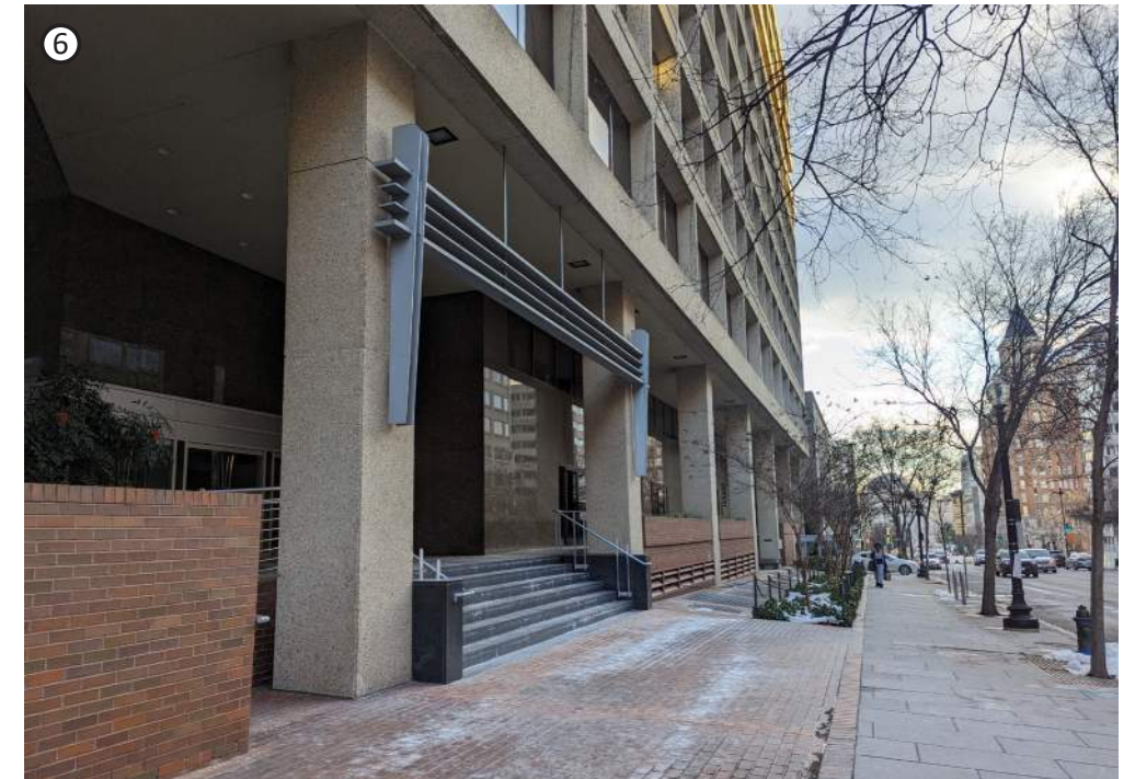
⑥ STEPS ON THE BACKSIDE OF THE BUILDING HAVE BEEN ALTERED TO MAKE ACCESS ADA COMPLIANT AND EXTEND THE ENTRANCE TOWARDS THE STREET
