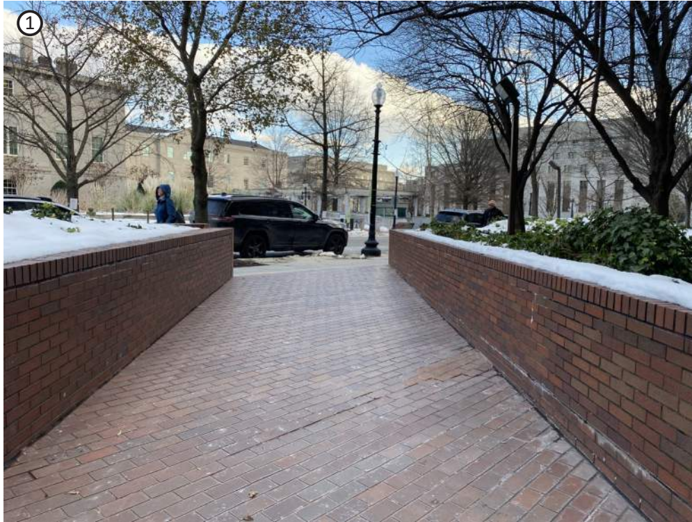
① BRICK WALLS BEND AT 45 DEGREE ANGLES TO WORK WITH DESIRED SIGHT LINES AND EASE OF ACCESS
