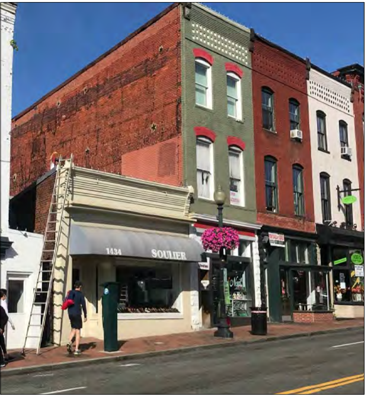
View from O street
