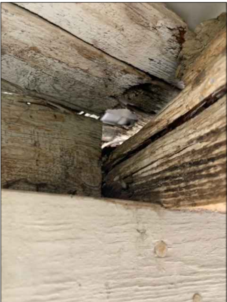
Existing Roof Framing Condition
