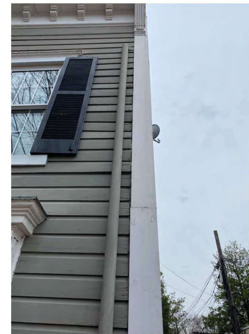
NORTHWEST CORNER SHOWING SIDING ROT FROM DOWNSPOUT
