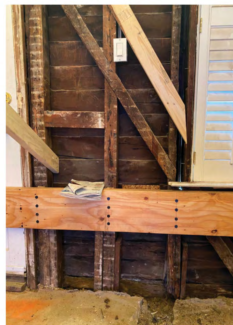
IMAGES DEPICTING EXISTING LAP SIDING FROM THE INTERIOR OF THE HOUSE - WE SUSPECT THAT THE MAJORITY IS SALVAGEABLE, EXCEPT FOR THE NORTH-WEST CORNER (TOP-TO-BOTTOM) AND THE VERY BOTTOM BELOW THE WINDOW SILLS
