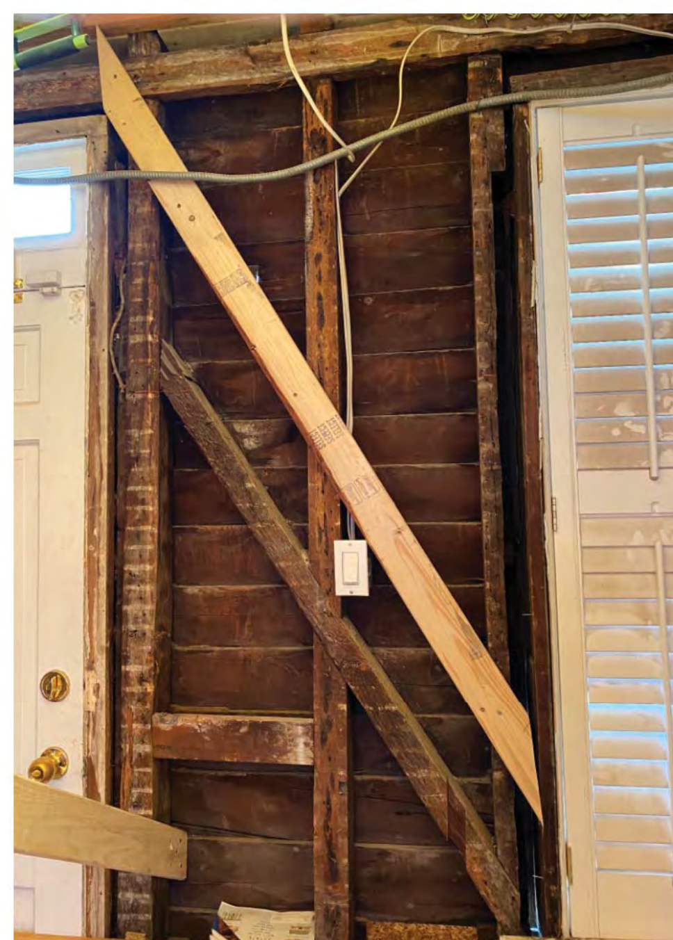
IMAGES DEPICTING EXISTING LAP SIDING FROM THE INTERIOR OF THE HOUSE - WE SUSPECT THAT THE MAJORITY IS SALVAGEABLE, EXCEPT FOR THE NORTH-WEST CORNER (TOP-TO-BOTTOM) AND THE VERY BOTTOM BELOW THE WINDOW SILLS
