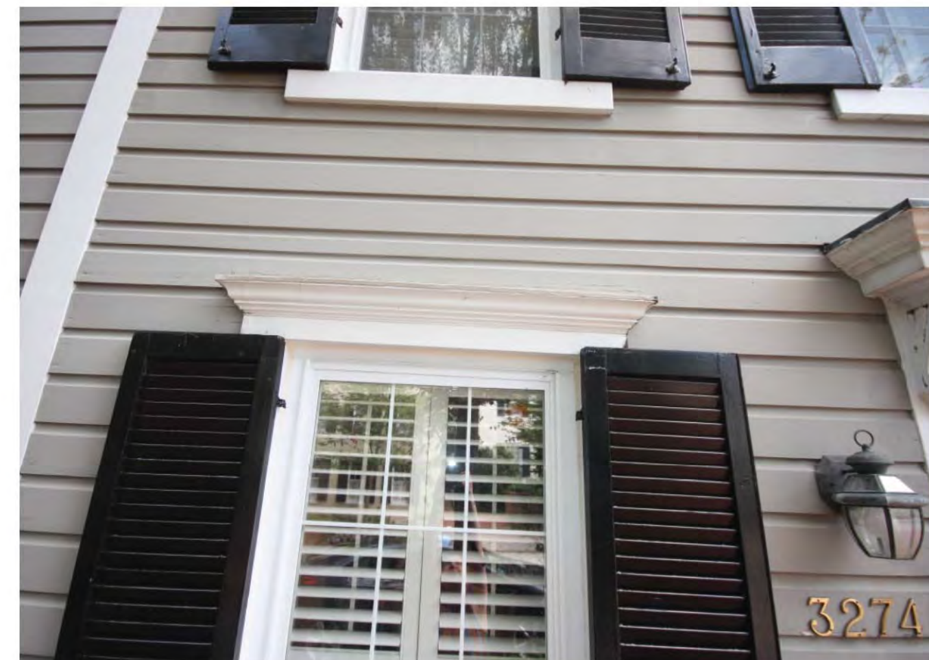
REPLACED HEAD TRIM AT FIRST FLOOR NORTH WINDOW
