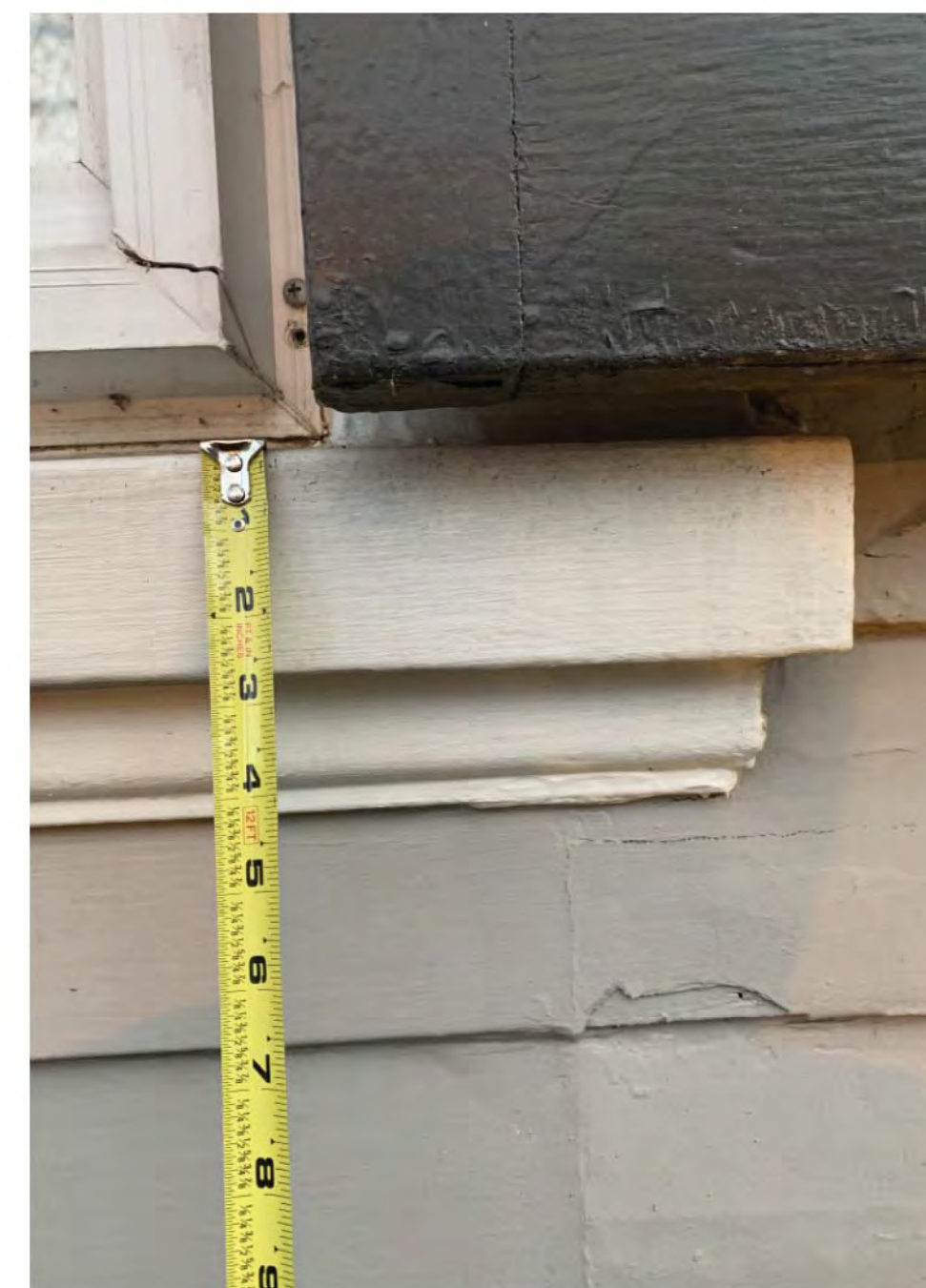
EXISTING WINDOW SILLS AT 3268 P STREET NW
