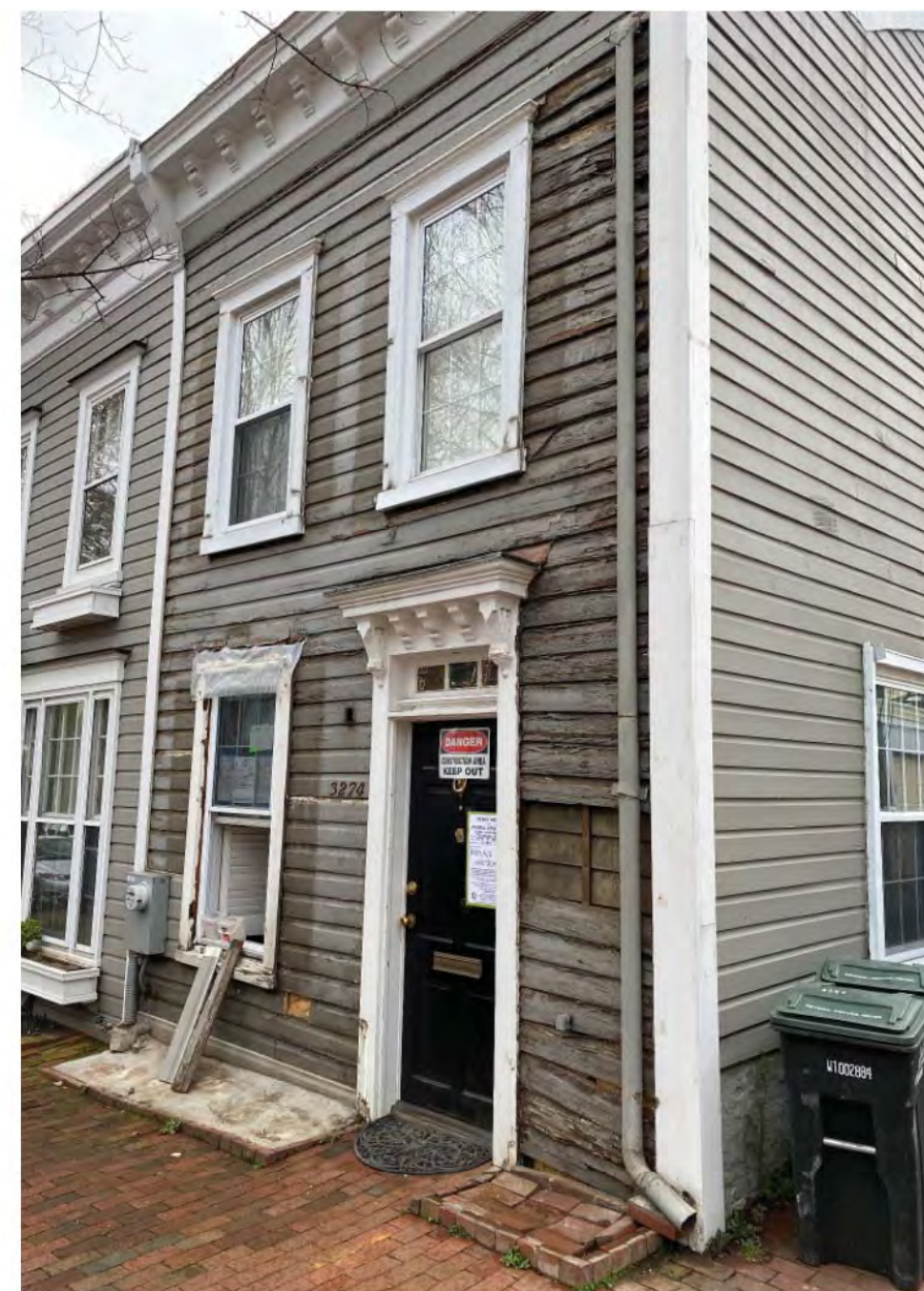
NORTH-WEST CORNER OF 3274 P STREET NW WITH FIRST OUTER LAYER OF SIDING REMOVED
