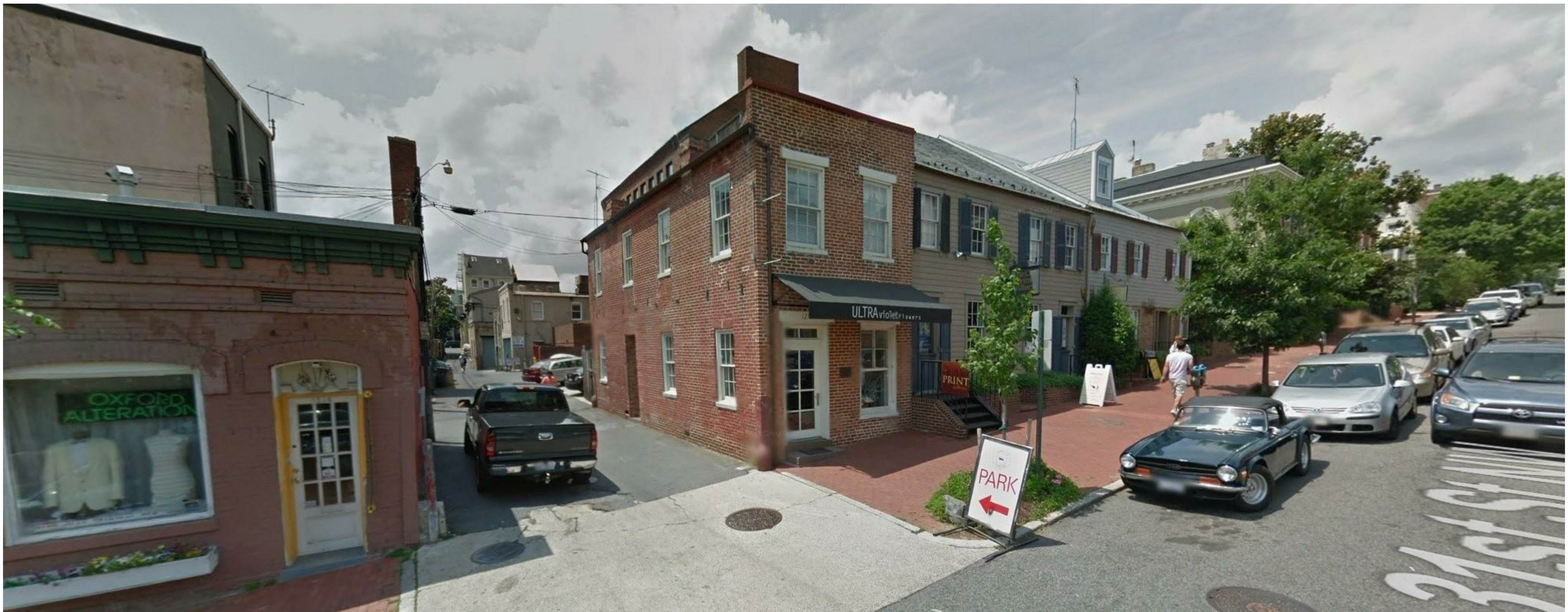
EXISTING STREET VIEW
