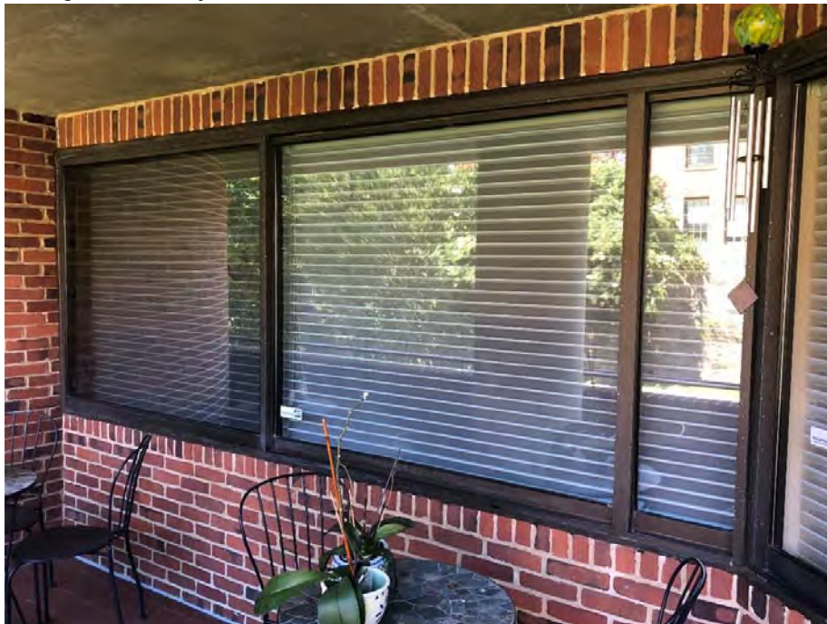
Sliding Window Adjacent to Door
