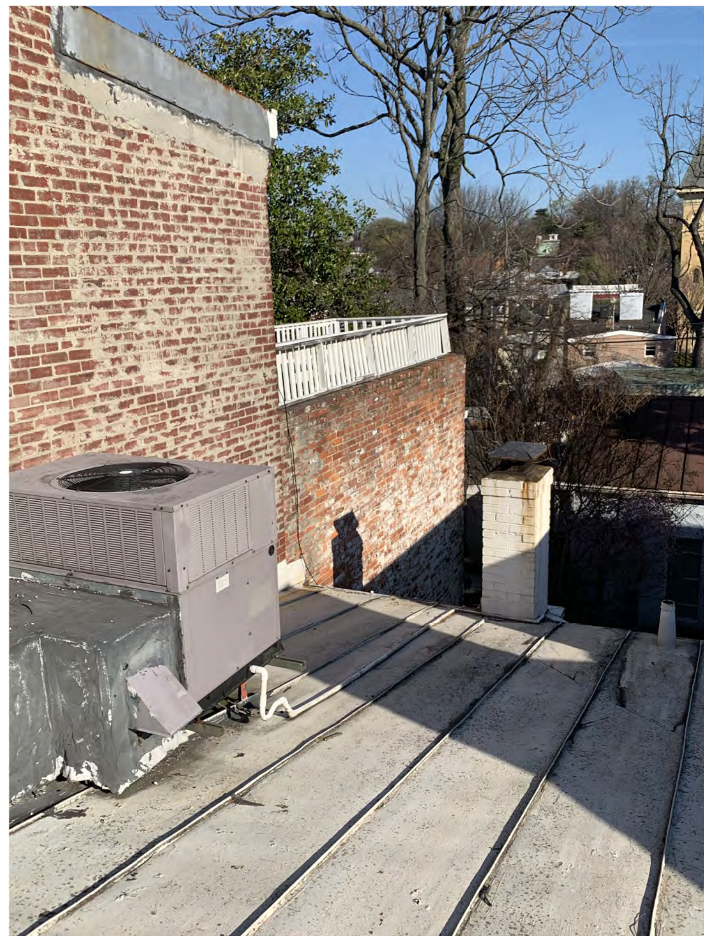
VIEW FROM ROOF LOOKING NORTHWEST
