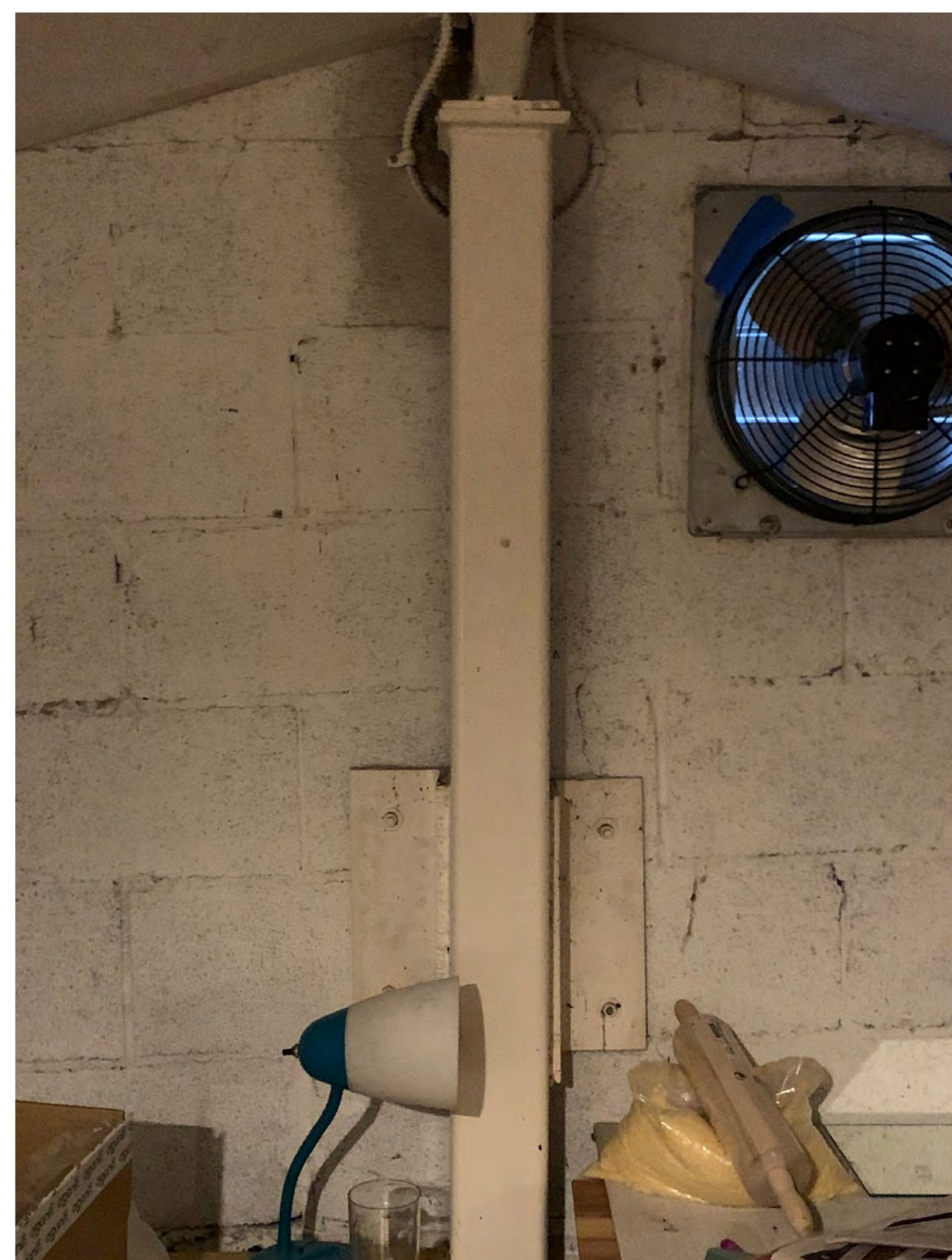
GARAGE LOFT INTERIOR WALLS W/ STEEL STRUCTURE
