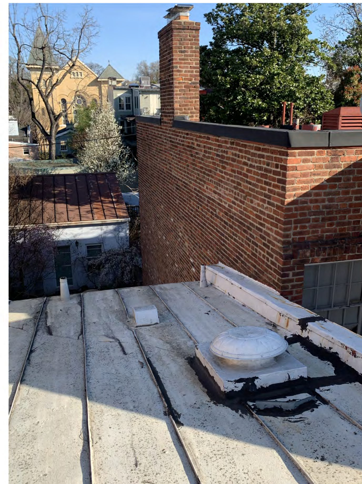
VIEW FROM ROOF LOOKING NORTHEAST
