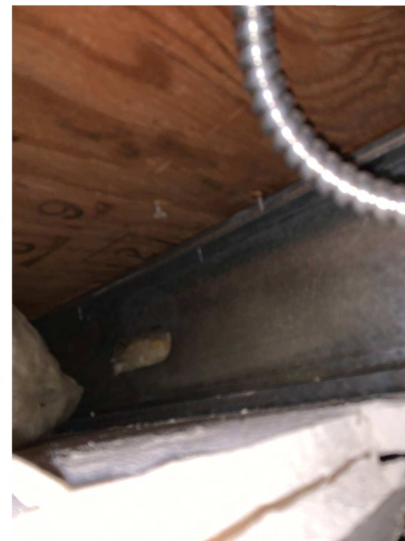
EXISTING GARAGE ROOF STRUCTURE: STEEL CHANNELS W/ PLYWOOD SHEATHING
