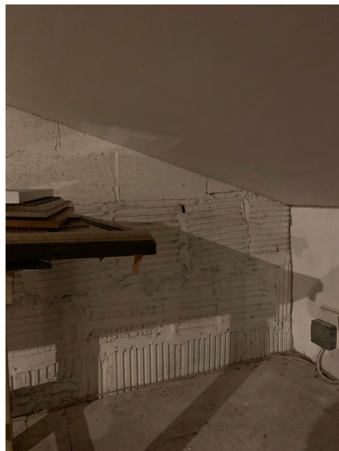
GARAGE LOFT INTERIOR WALLS: TERRA COTTA BLOCK W/ CMU ABOVE
