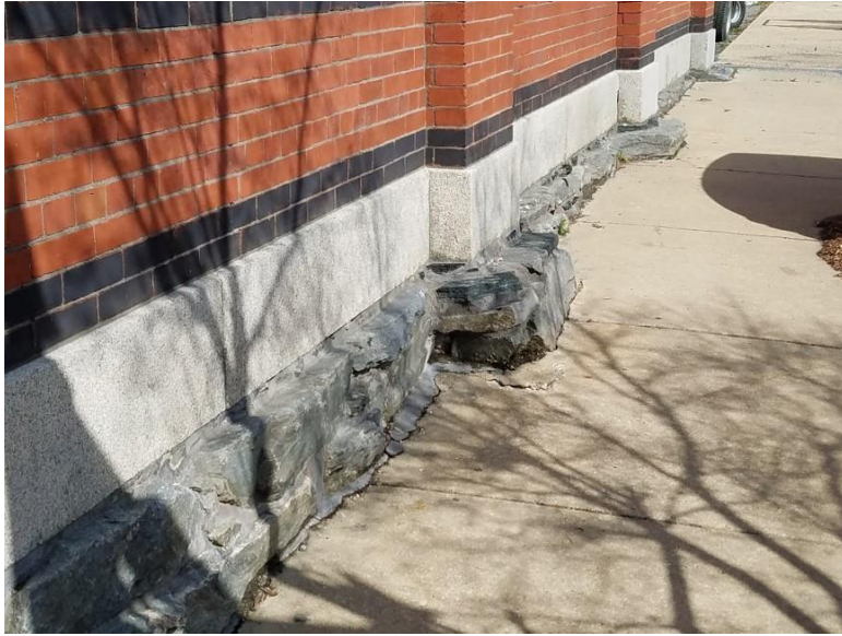
Exposed AIB gneiss foundation - east elevation at South corner.
