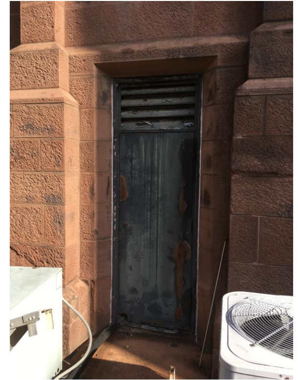
Existing window in south areaway converted to a door.
