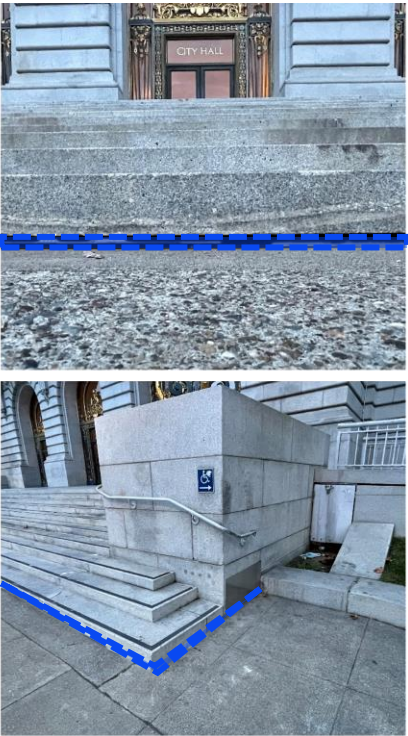
Integrated seismic joint cover examples.
