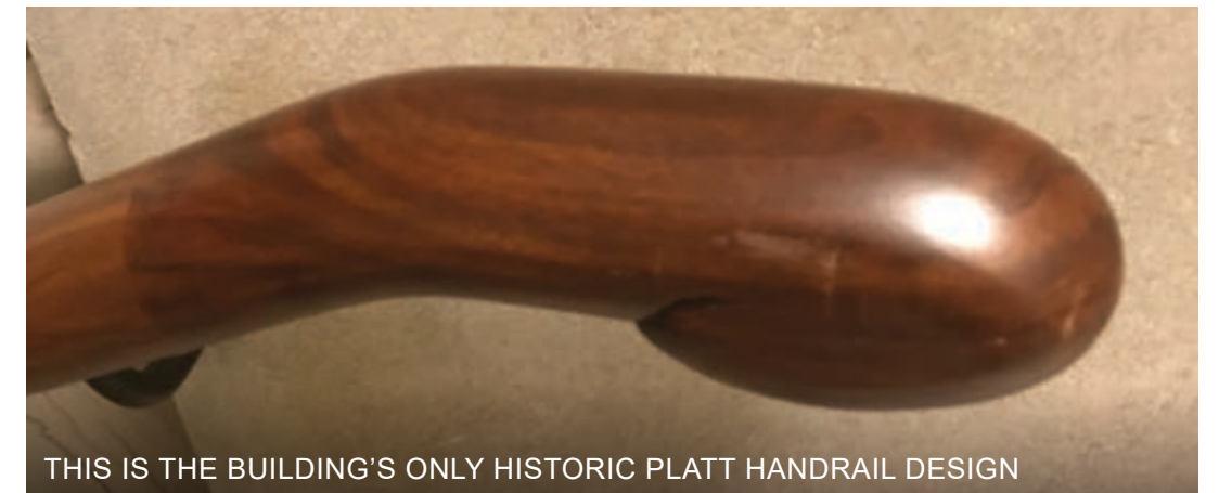
EXISTING INTERIOR HANDRAIL
