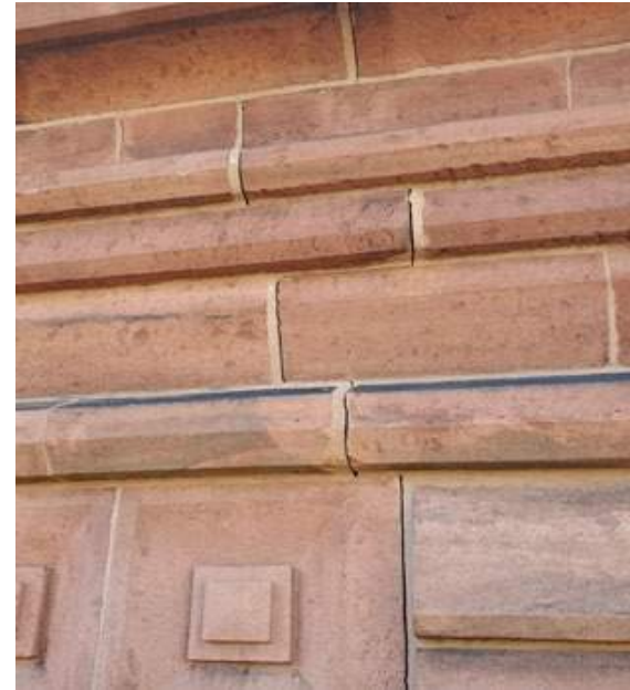
Existing Cracked Masonry
