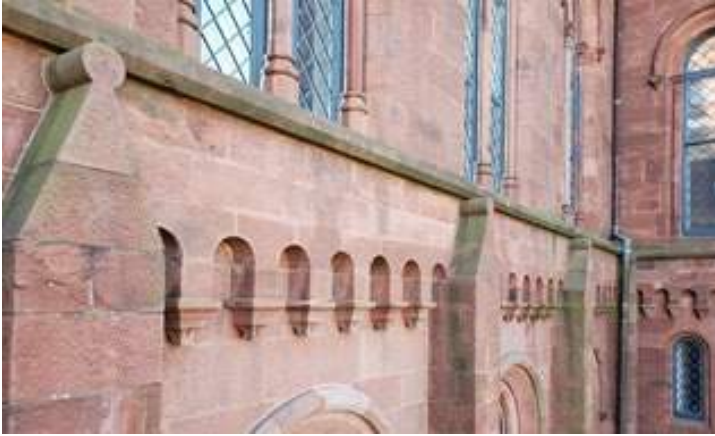
Biological Growth Staining Concentrated at Horizontal Projections
