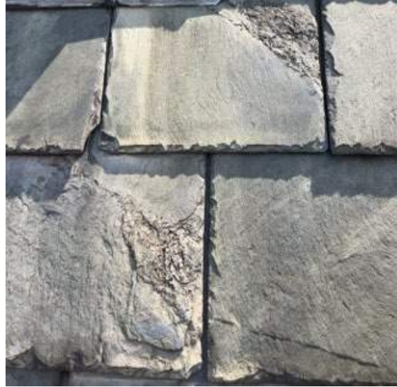
Typical Deterioration of Slate Shingles
