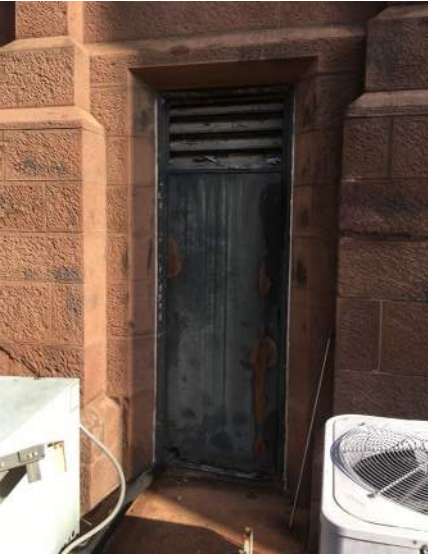
Window in South Areaway Converted to a Door
