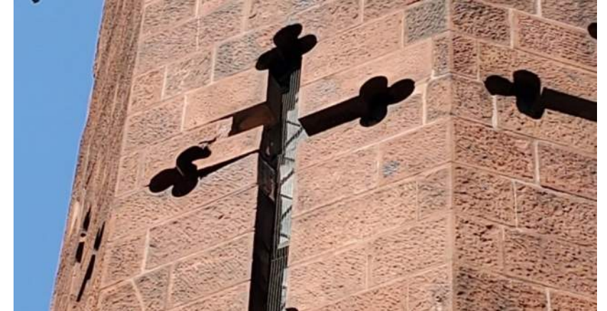
Loose Stone on Octagon Tower (Has Since Been Removed)
