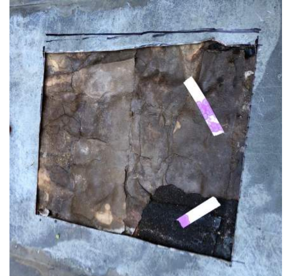
Water Below Copper Roofing, Typical
