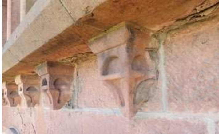
Masonry Damage Below Horizontal Projections
