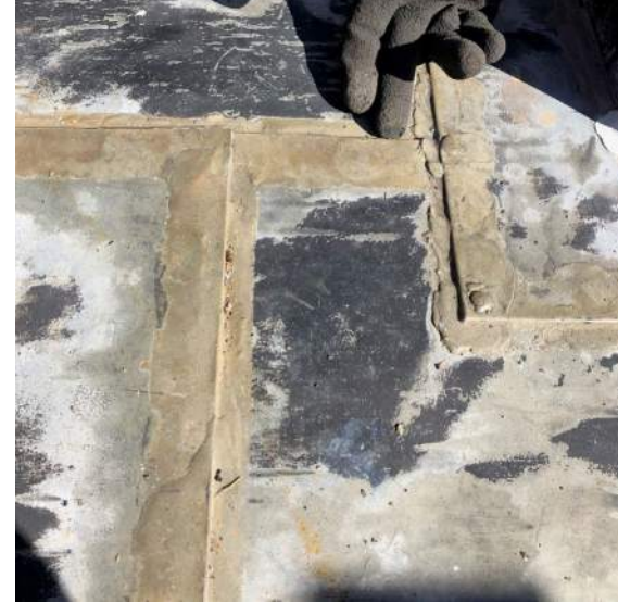
Typical Thin Solder at Seams in Copper Seams
