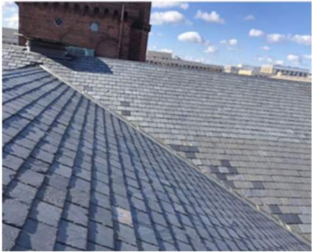
Typical Slate Roofing
