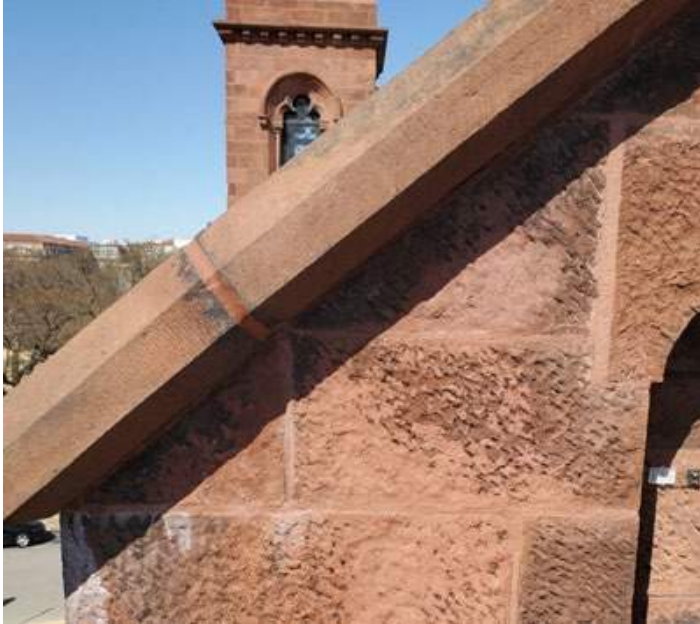
Previous Repairs on Masonry, Including Sealant in Joints and Surface-Applied Mortar Repairs
