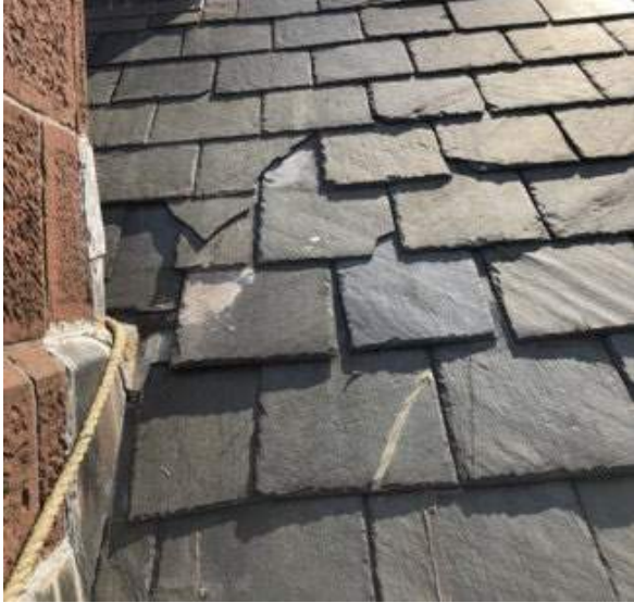
Typical Broken, Missing, or Loose Slate Shingles
