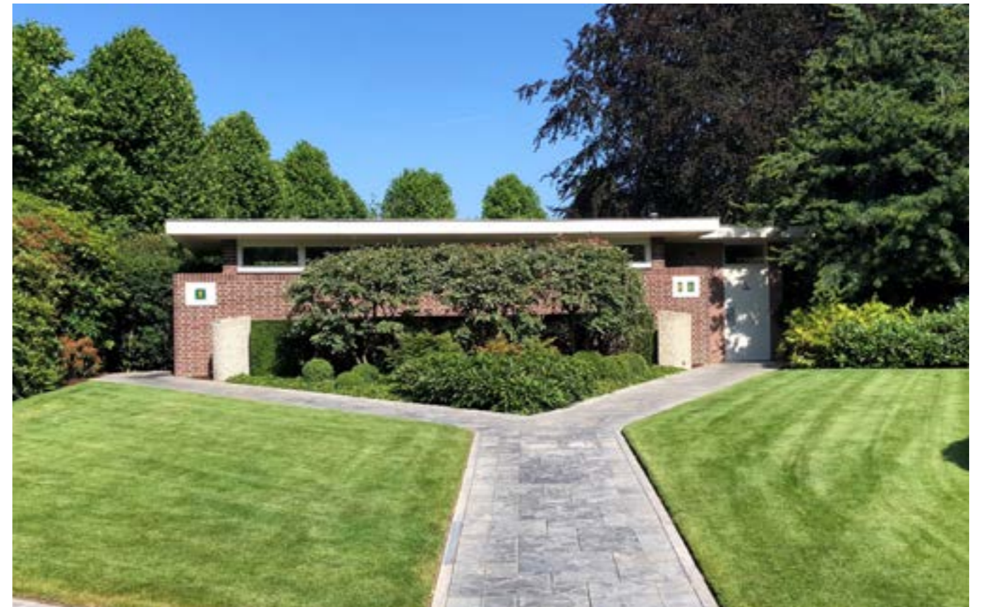
Restroom facility in 2019
