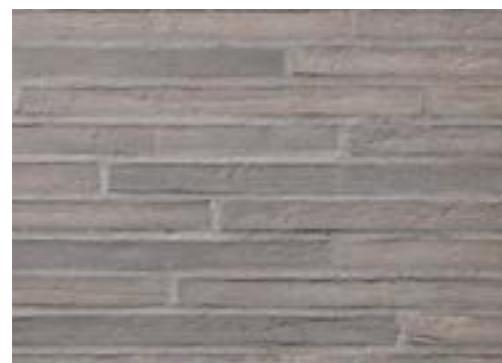
walls + floor exterior:
