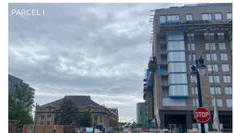
WASA PUMPING STATION IN RELATION TO PARCEL I (110')
