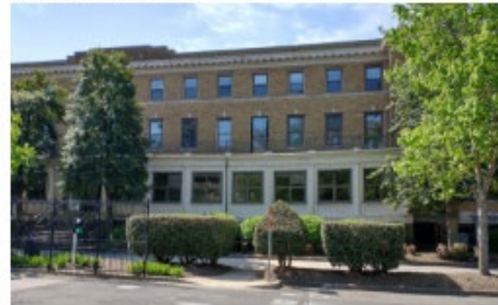
NORTH PORCH OF B166
