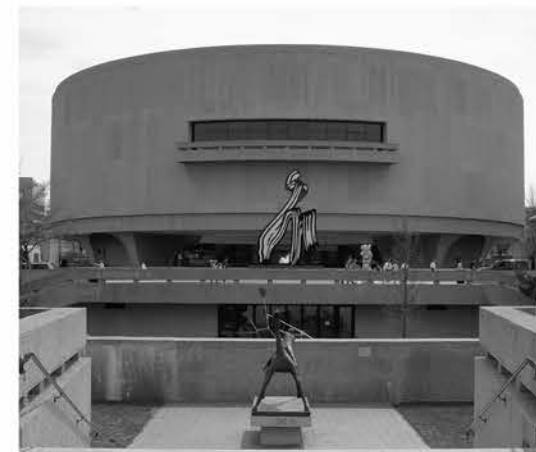
Third -Story Balcony and Fenestration
