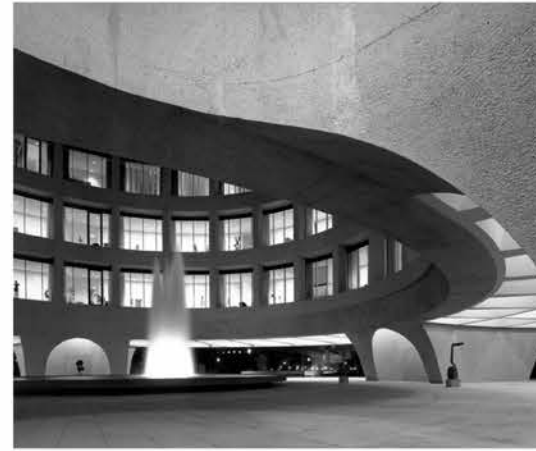
Sculptural, Cast-In-Place Concrete Piers
