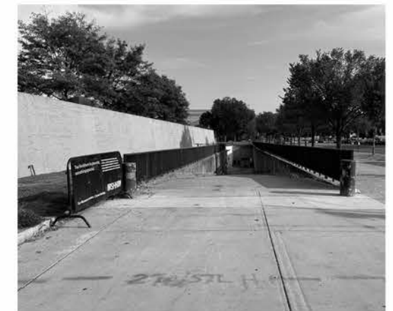
Loading Dock Ramp, Retaining Walls, & Fence
