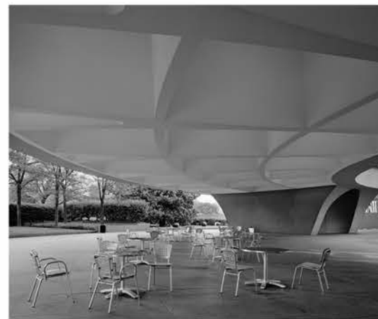
Painted, Coffered Concrete Ceiling
