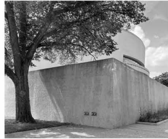
Battered Perimeter Walls
