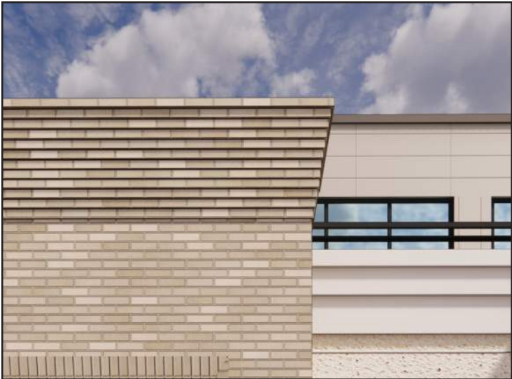
A: Brick Corbeling at the Top of the Bays
