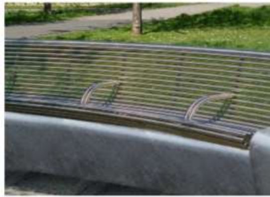
18" GRANITE WALL WITH INSERTED MODULAR STEEL SEATING (ADA COMPLIANT)
