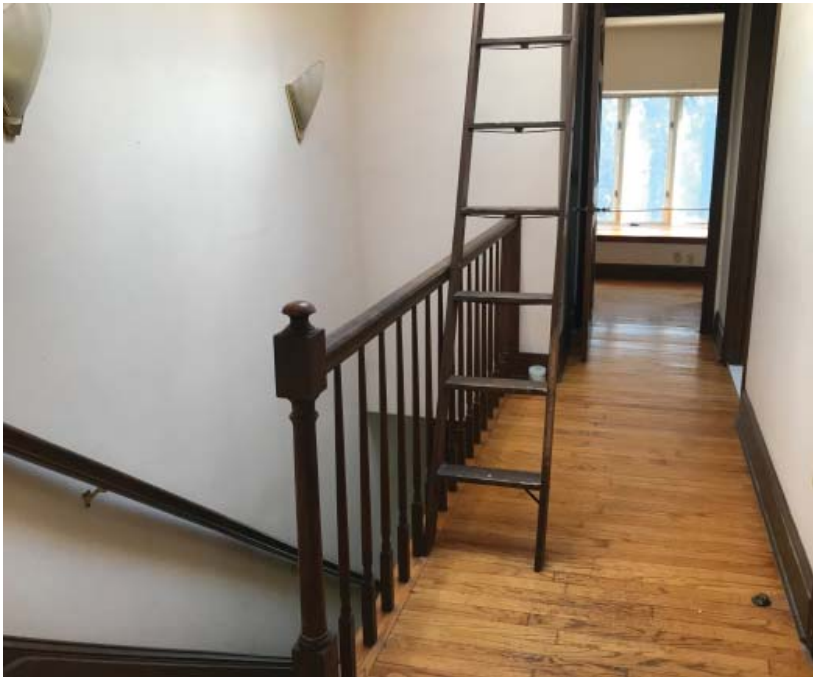
VIEW OF SECOND FLR STAIR HALL
