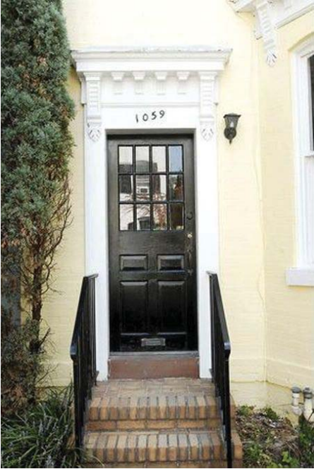
4 1059 THOMAS JEFFERSON ST. NW PREVIOUS EXTERIOR WEST ENTRY
