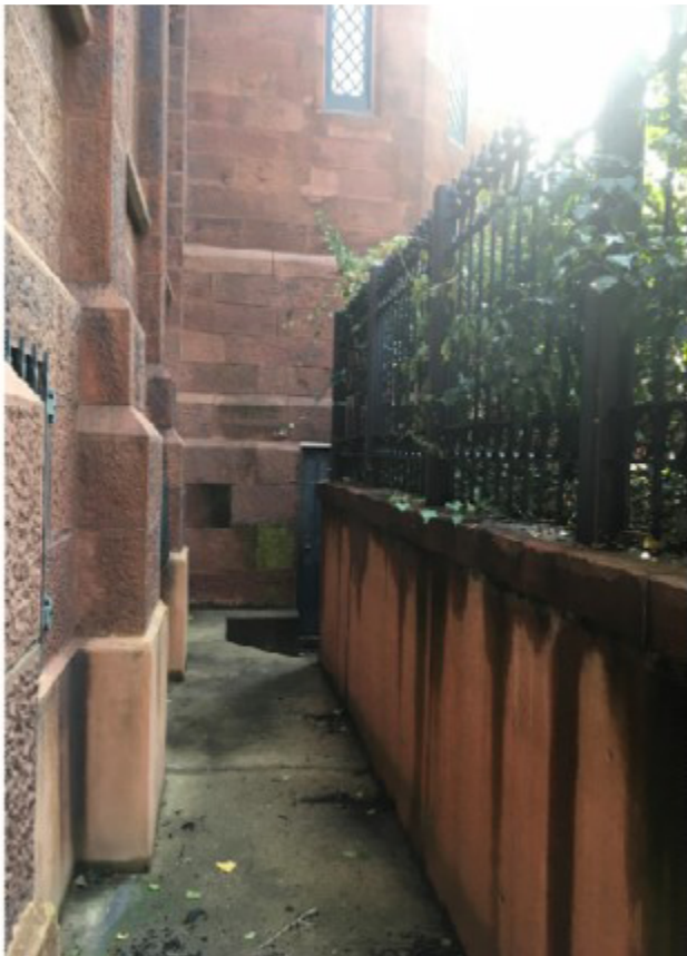
Figure 3.1.2.b - Existing character of south areaways
