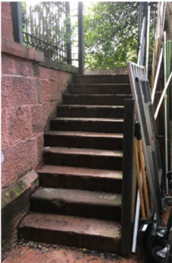
Figure 3.1.2.d - Existing character of south areaways
