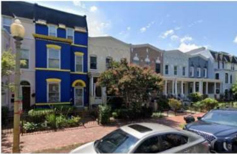
Row Houses on L St
