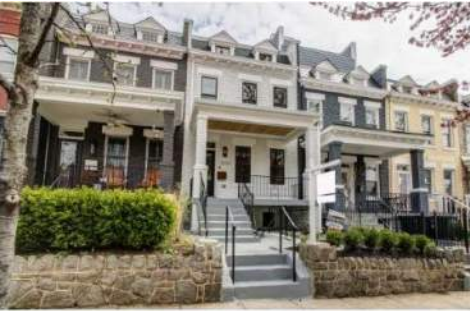
Row Houses on 7 th St
