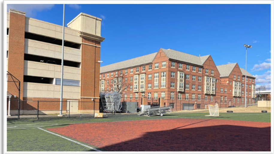
View of K Street Security Gate
