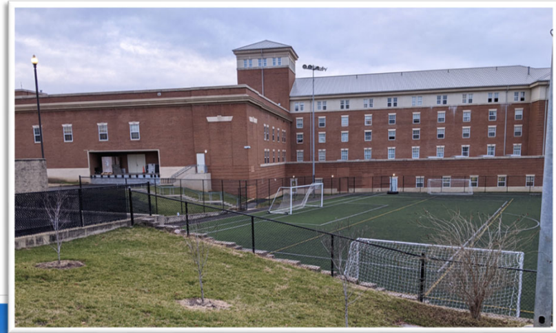
View of Existing Building 25 Tower
