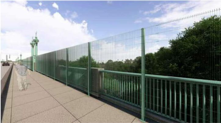
Rendering at railing and typical pilasters
