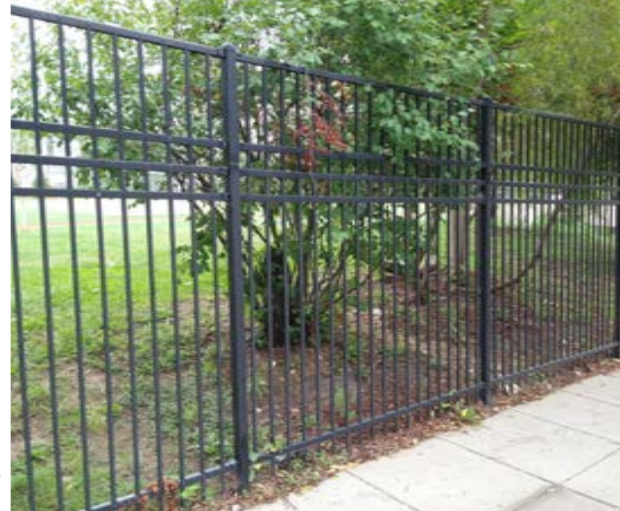
1. DPR PERIMETER FENCE
