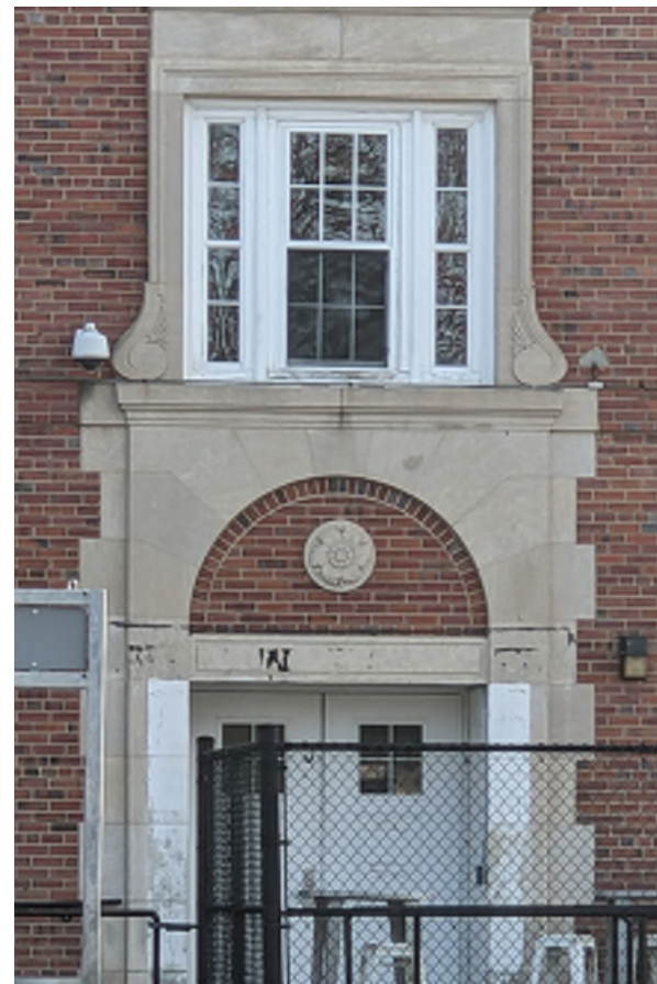
Historic Cast Stone on West Facade
