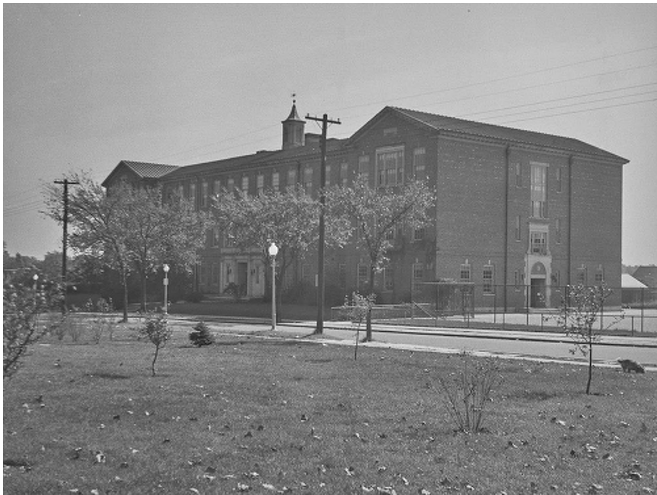
Historic School Building, ca. 1948, showing 12 over 12 lites in windows
