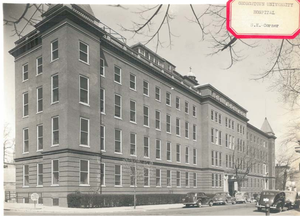
1. LOYOLA HALL SOUTH-EAST ELEVATION - 1944
