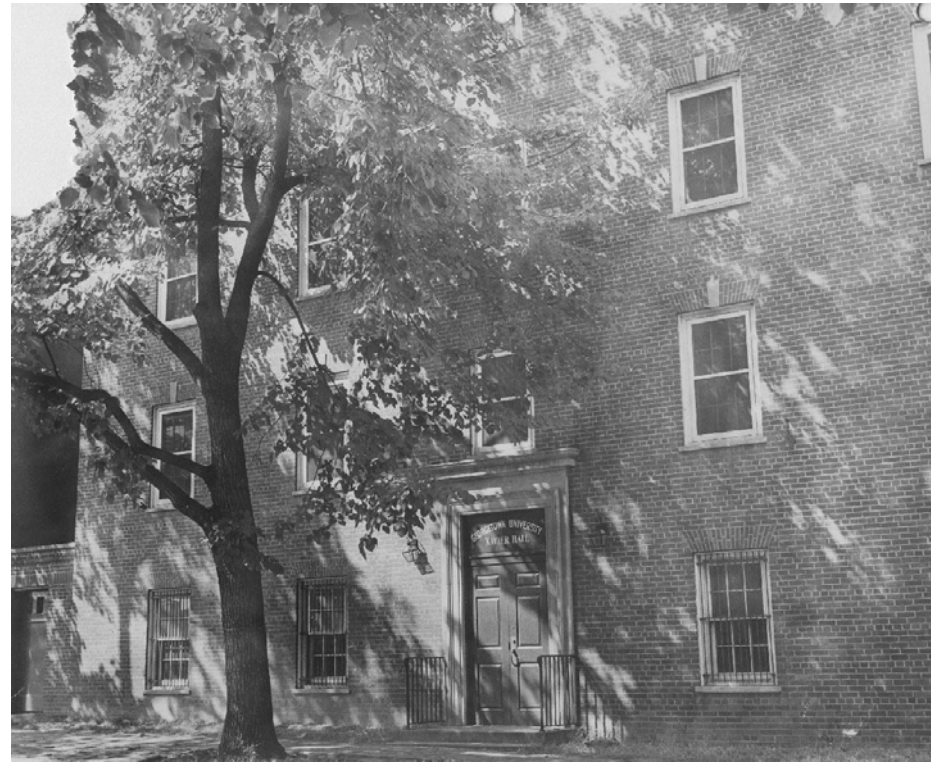
2. XAVIER HALL SOUTH-WEST ELEVATION - PROSPECT STREET - 1956
