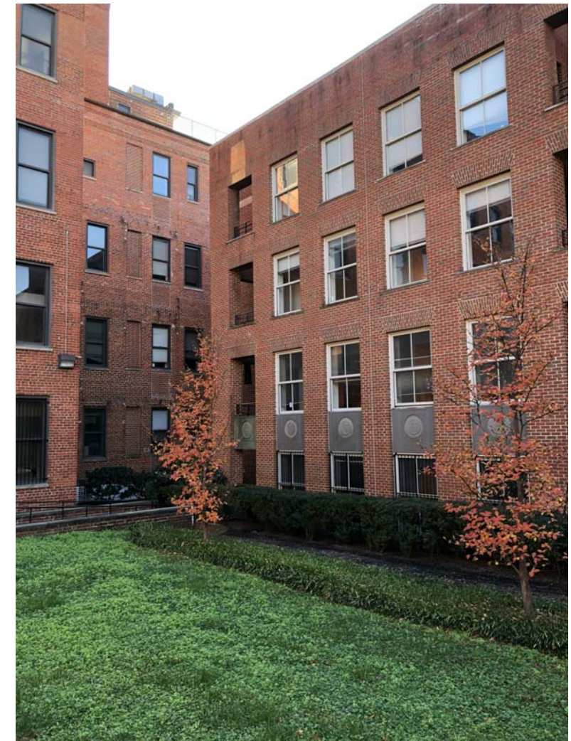
3. XAVIER HALL NORTH ELEVATION
