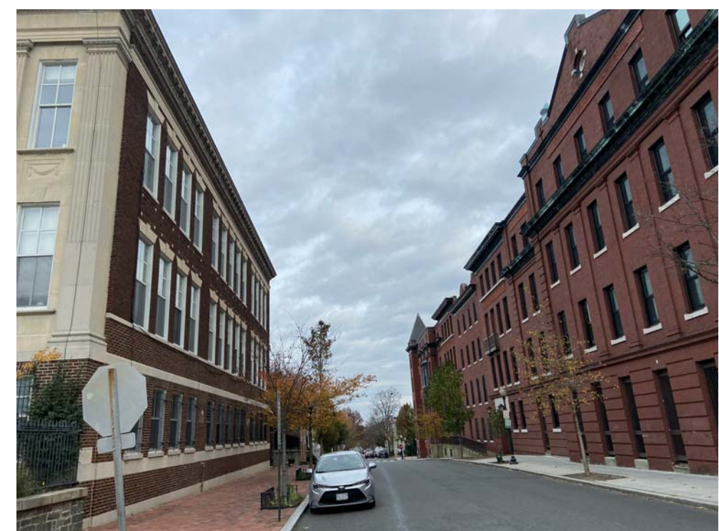
5. LOYOLA HALL - N STREET NORTH - WEST
