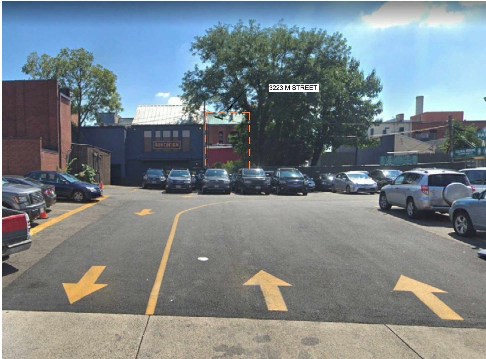
REAR VIEW - PROSPECT STREET
