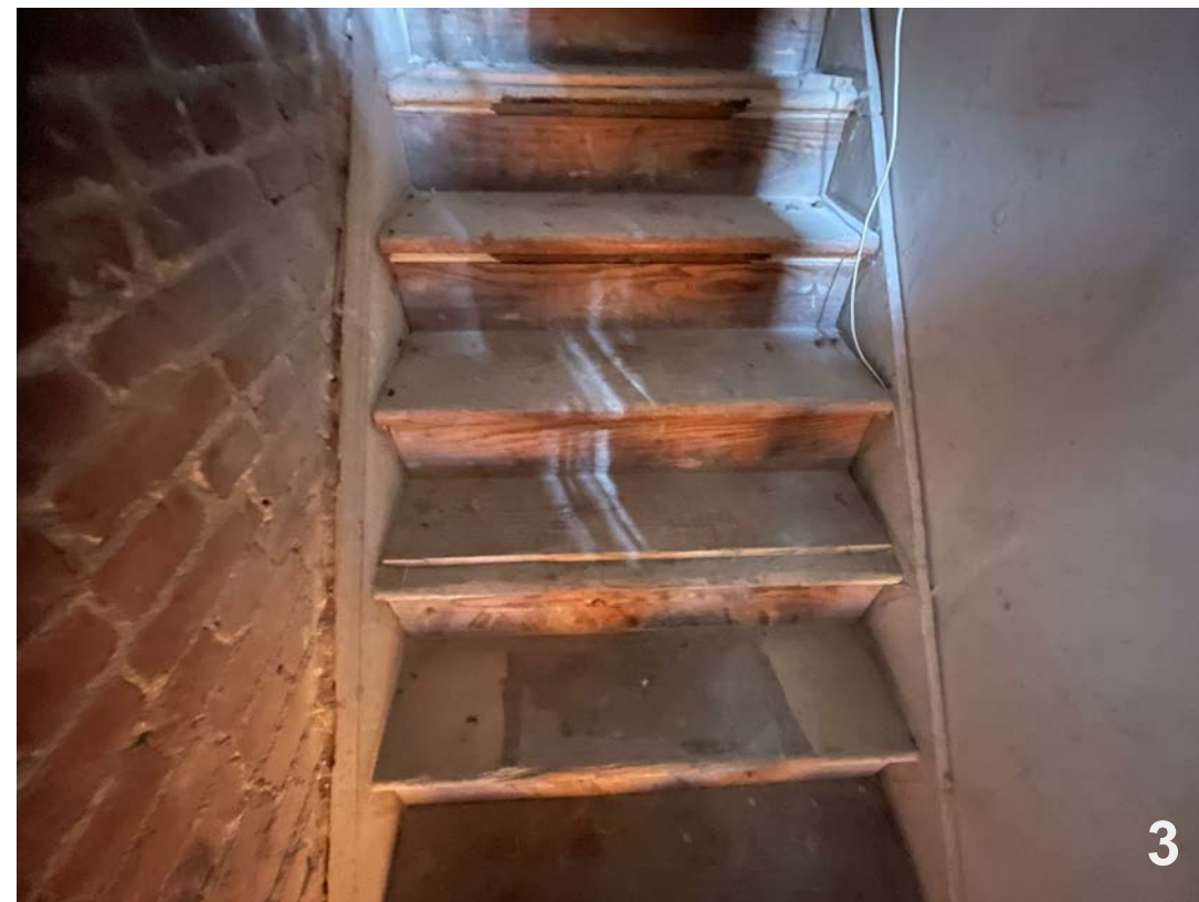
STAIRS FROM GROUND LEVEL TO LEVEL TWO. METAL PLATFORM WITH ATTACHED BANISTER AN NON CODE COMPLIANT STAIRS
