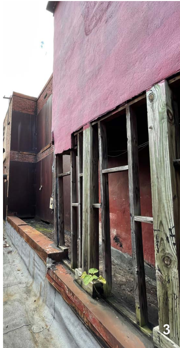
EXISTING EAST ELEVATION PARTY WALL WINDOWS COVERED WITH STEEL PLATES
