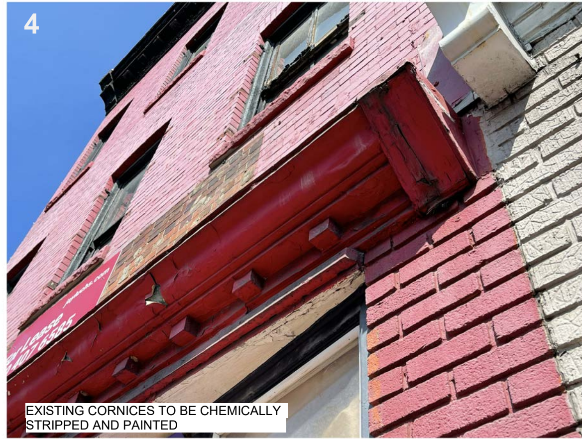
EXISTING CORNICES TO BE CHEMICALLY STRIPPED AND PAINTED
