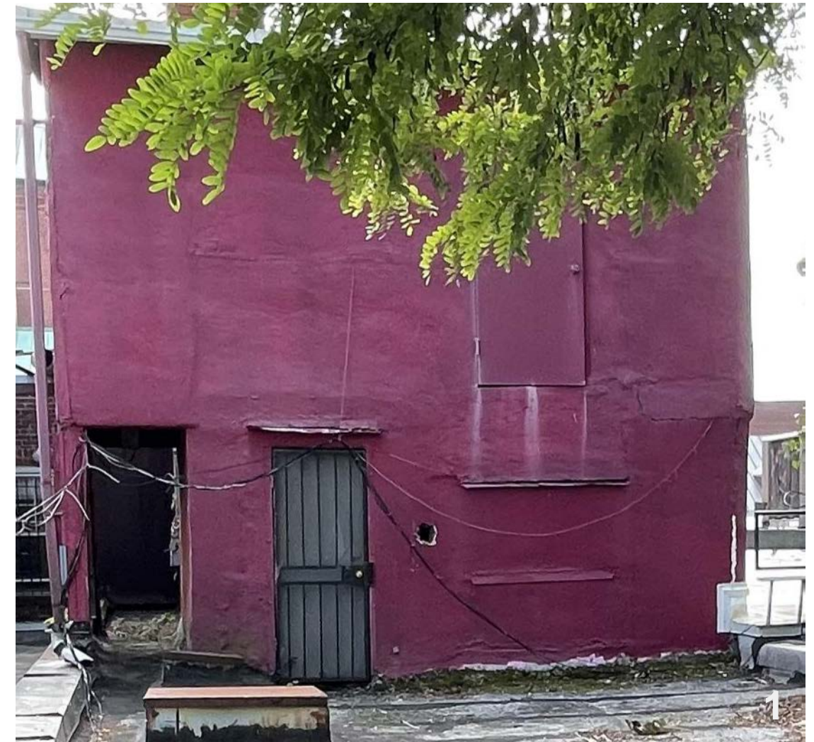
EXISTING REAR ELEVATION. NON HISTORIC DOORS AND PLASTER/WOOD WALLS
