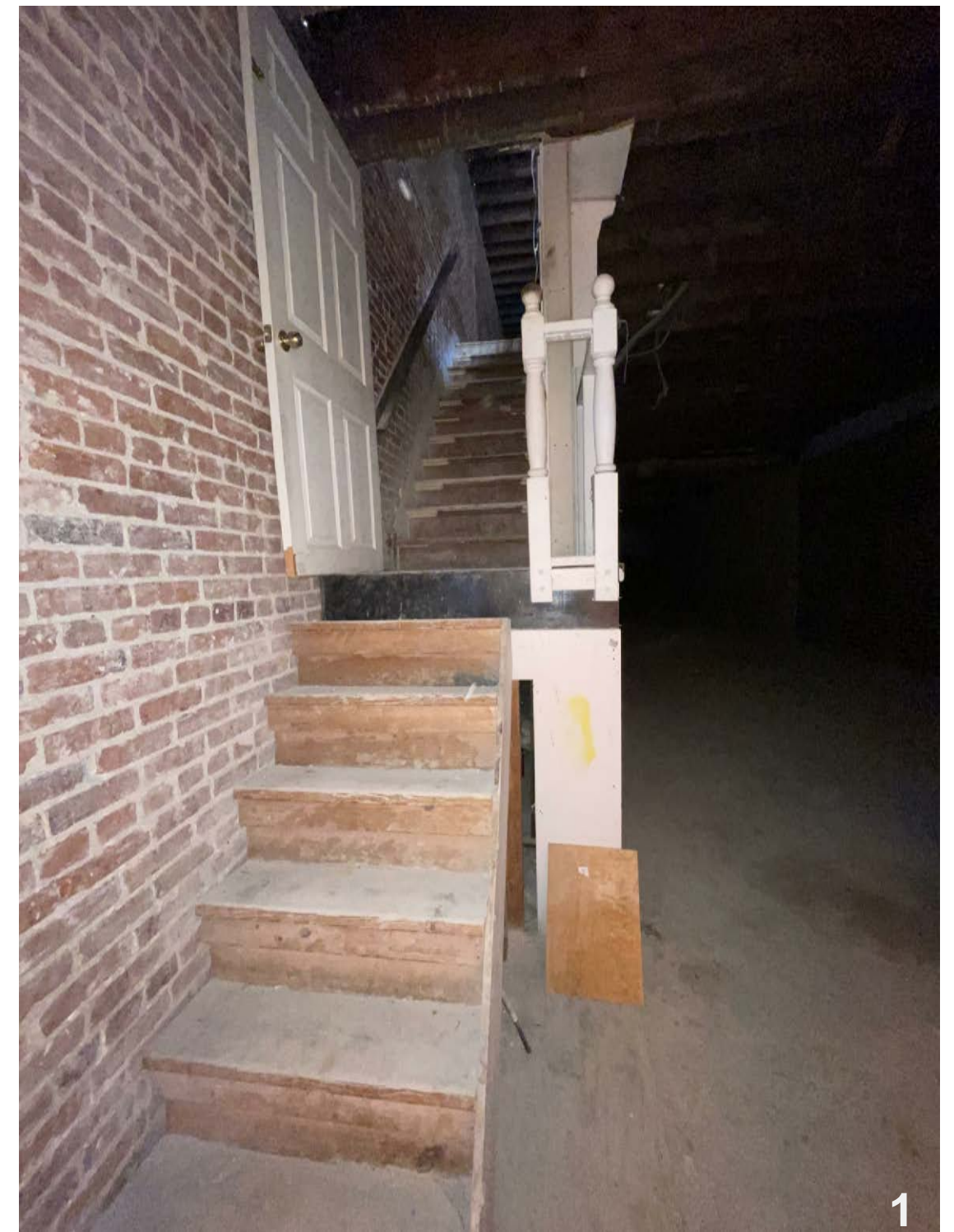
STAIRS FROM GROUND LEVEL TO LEVEL TWO. METAL PLATFORM WITH ATTACHED BANISTER AN NON CODE COMPLIANT STAIRS
