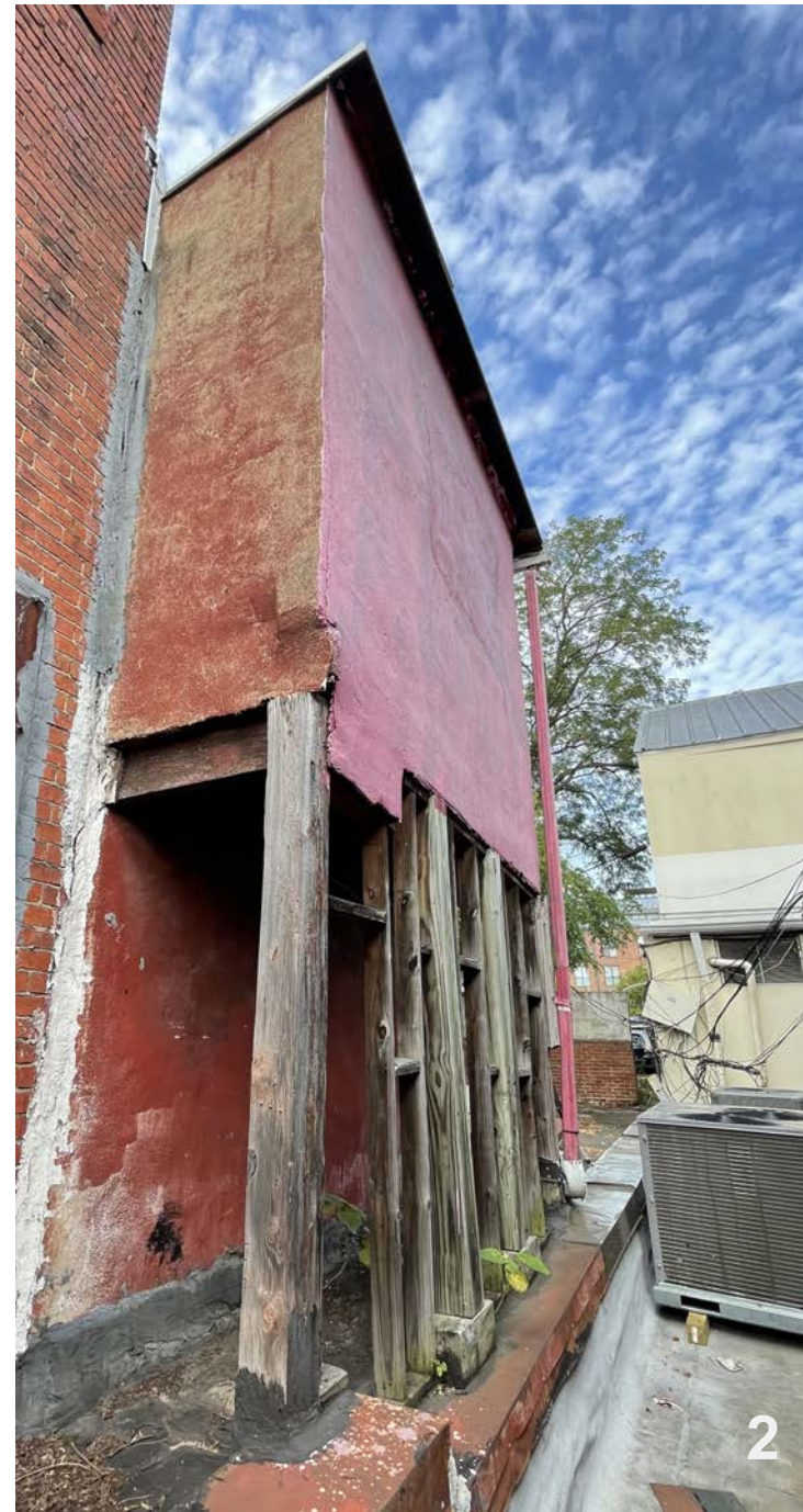
REAR ADDITION - PLASTER WALLS / NO BRICK -NON HISTORIC. STRUCTURE IN BAD STATE AND NON- CODE COMPLIANT
