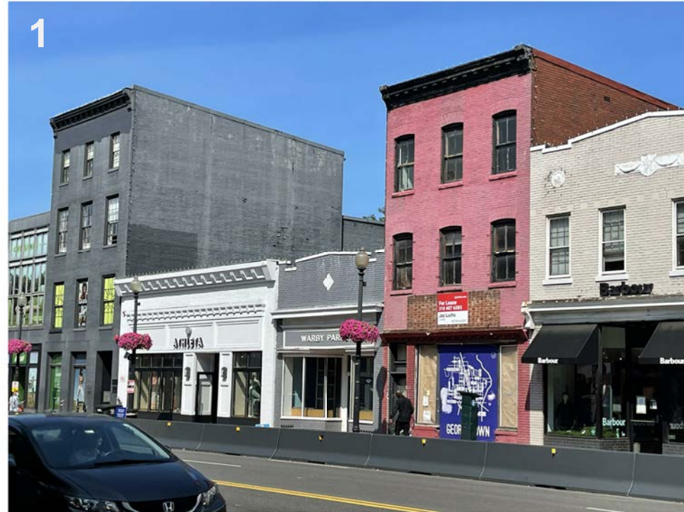
EXISTING CORNICES TO BE CHEMICALLY STRIPPED AND PAINTED
