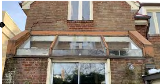
5A EXISTING CONDITION IMAGE - MASONRY CRACK
