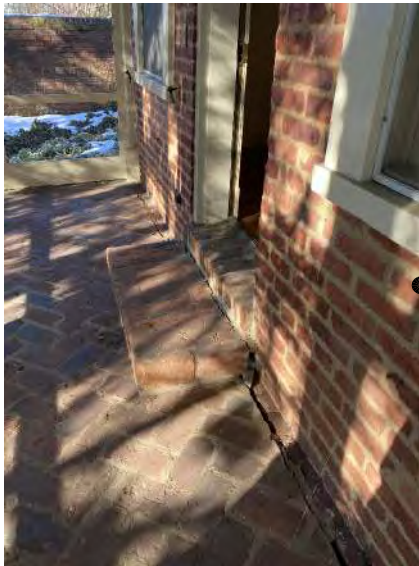
2A EXISTING CONDITION IMAGE - FROST HEAVE
