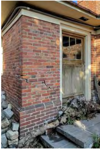
4A EXISTING CONDITION IMAGE - MASONRY CRACK
