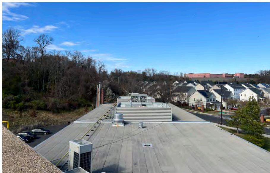
East Wing Roof
