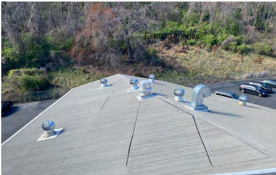
Site to North from Roof
