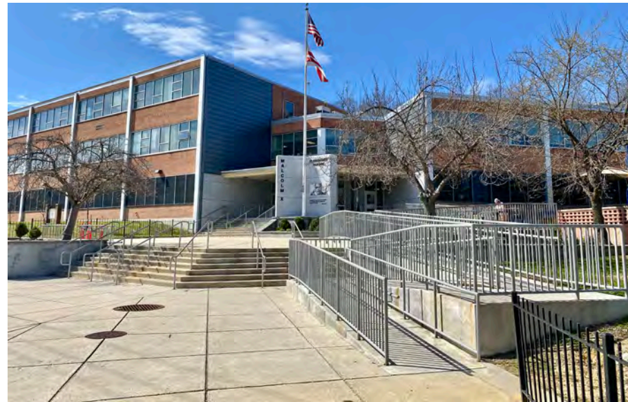
Main Building Entrance from Mississippi Avenue
