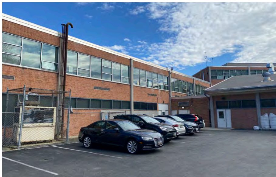
East Wing Rear Elevation
