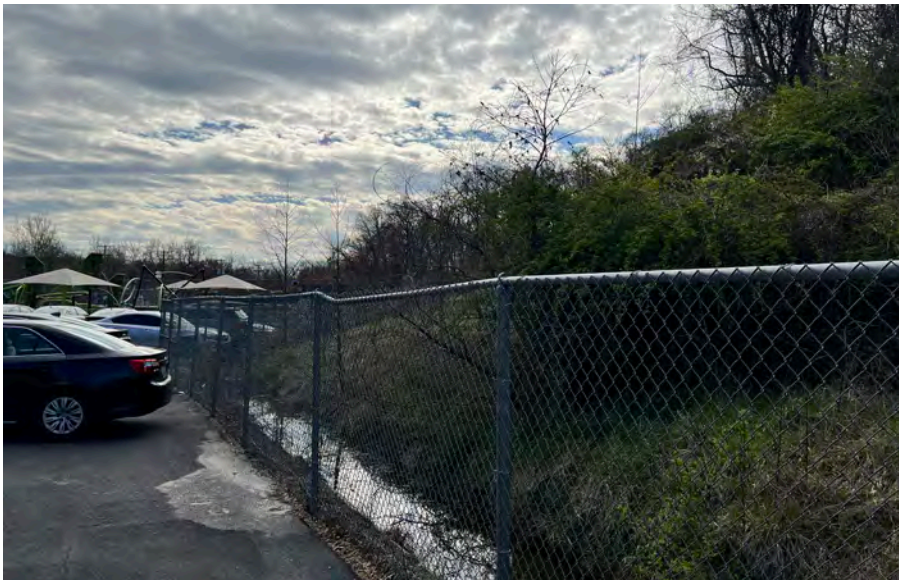
North Hillside and Site Gutter
