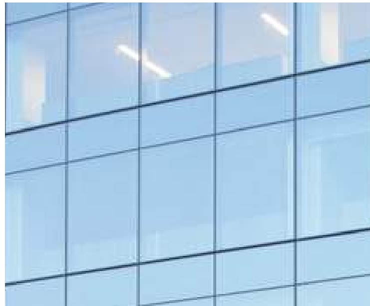
NEW CURTAIN WALL
