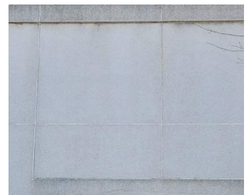
EXISTING PRECAST on existing window sill and head
