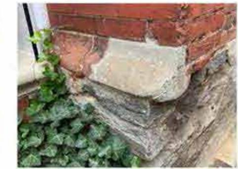
Restore, or replace damaged bricks above stone base
