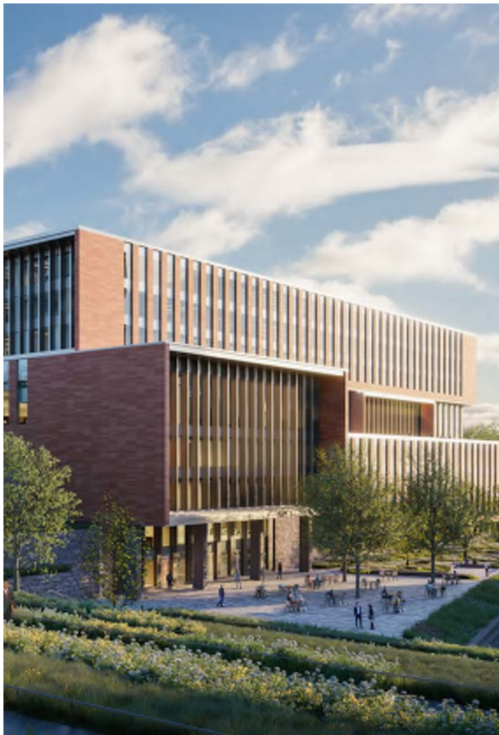
B1 CISA (IN PROGRESS)
