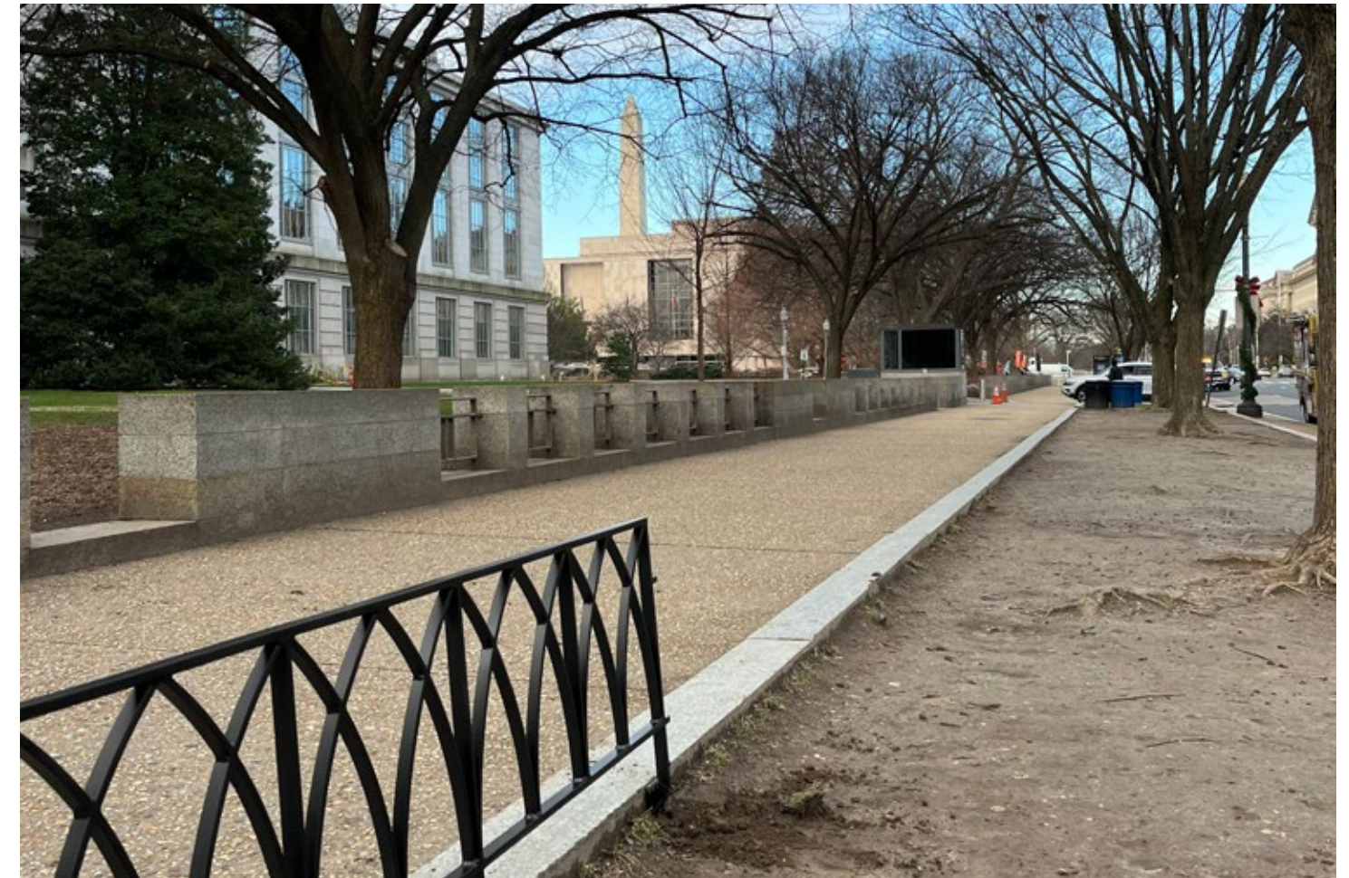
North Elevation, looking southeast Constitution Avenue NW at NMNH
