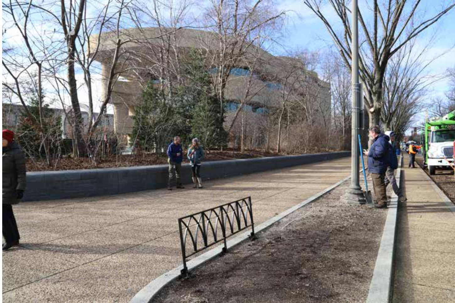
Northeast Elevation, looking southwest Jefferson Drive SW at NMAI
