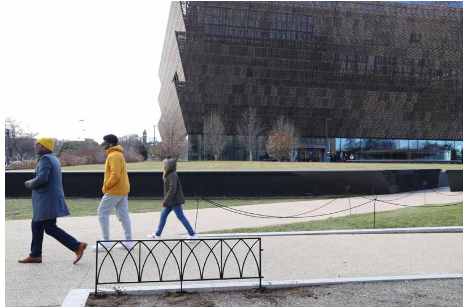
North Elevation, looking south Constitution Avenue NW at NMAAHC
