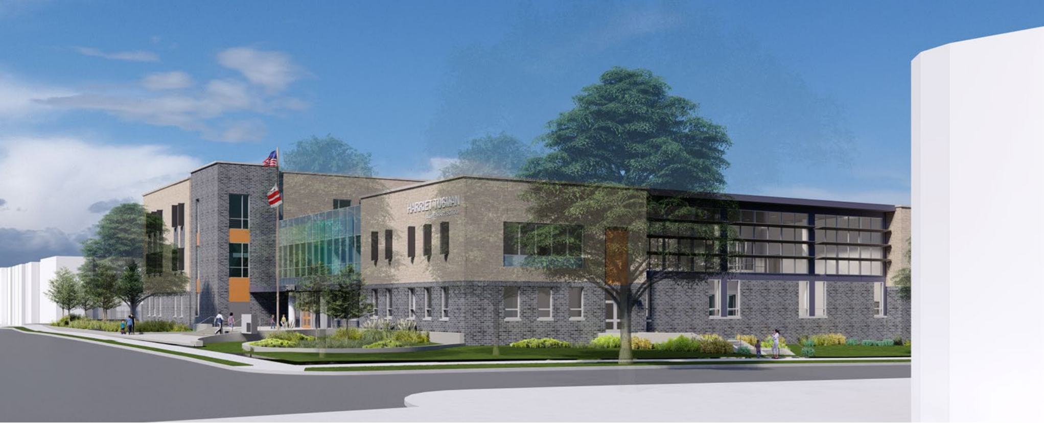
View – Corner of 13th St and Irving St looking north
