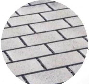
PERMEABLE CONCRETE PAVERS (PARKING SPACES)
