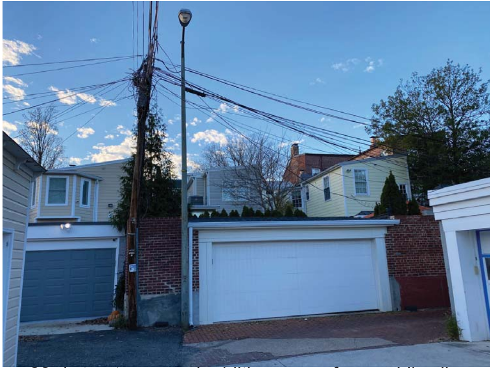
a - 33rd street rear yard additions seen from public alley
