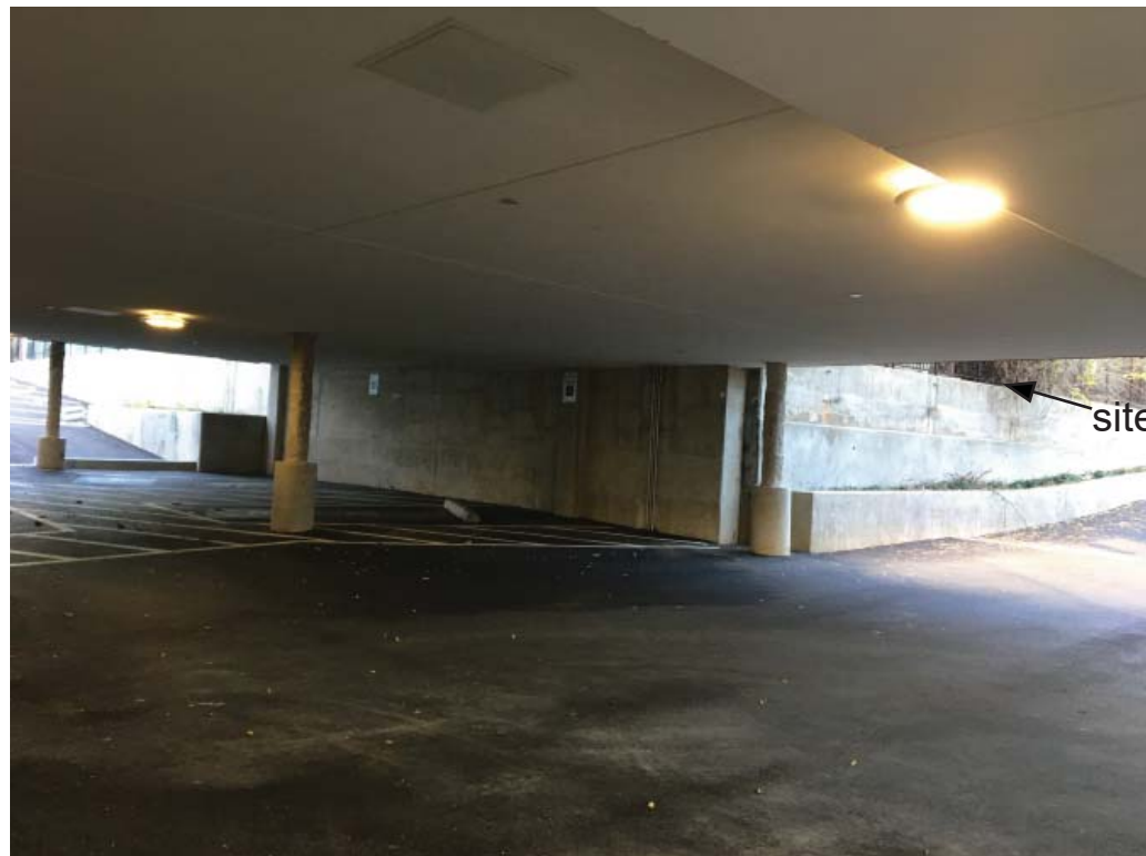
view from parking structure, towards rear of site
