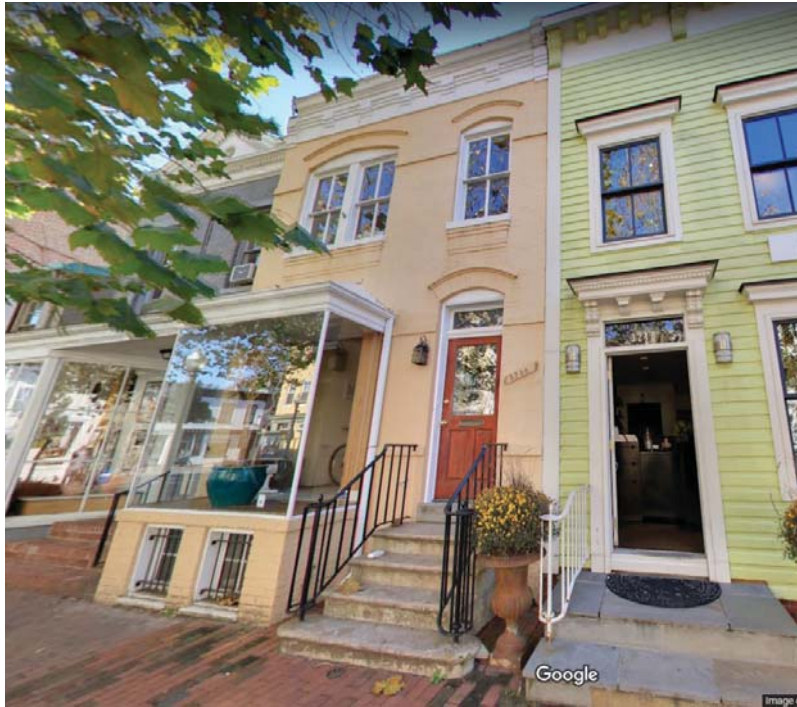
front facade, previous colors, seen from p street
