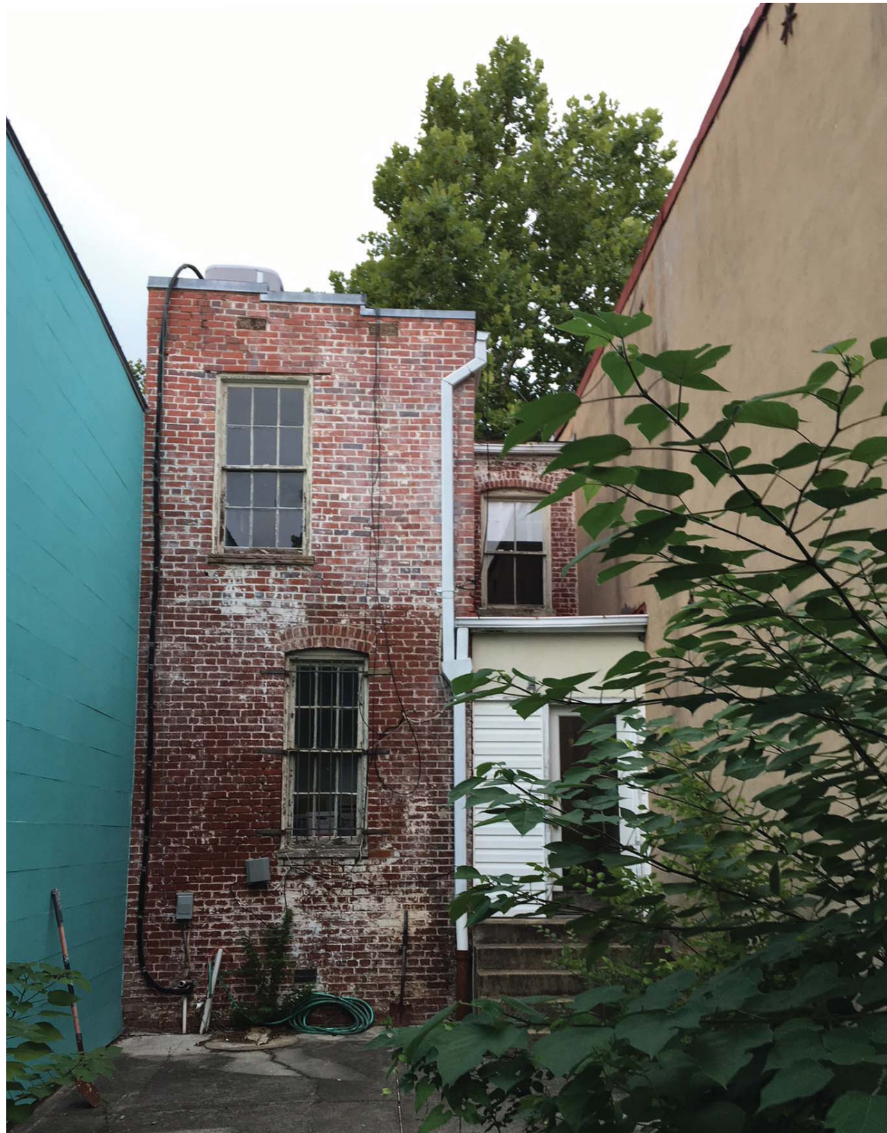
existing rear facade
