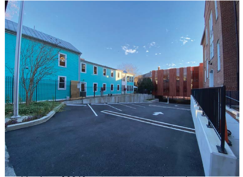
c - side view of 3240 p street nw, seen through gate
