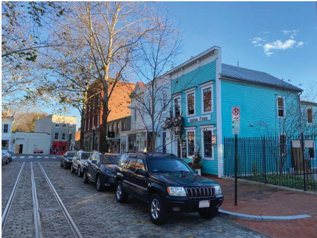
front facade in context, west on p street
