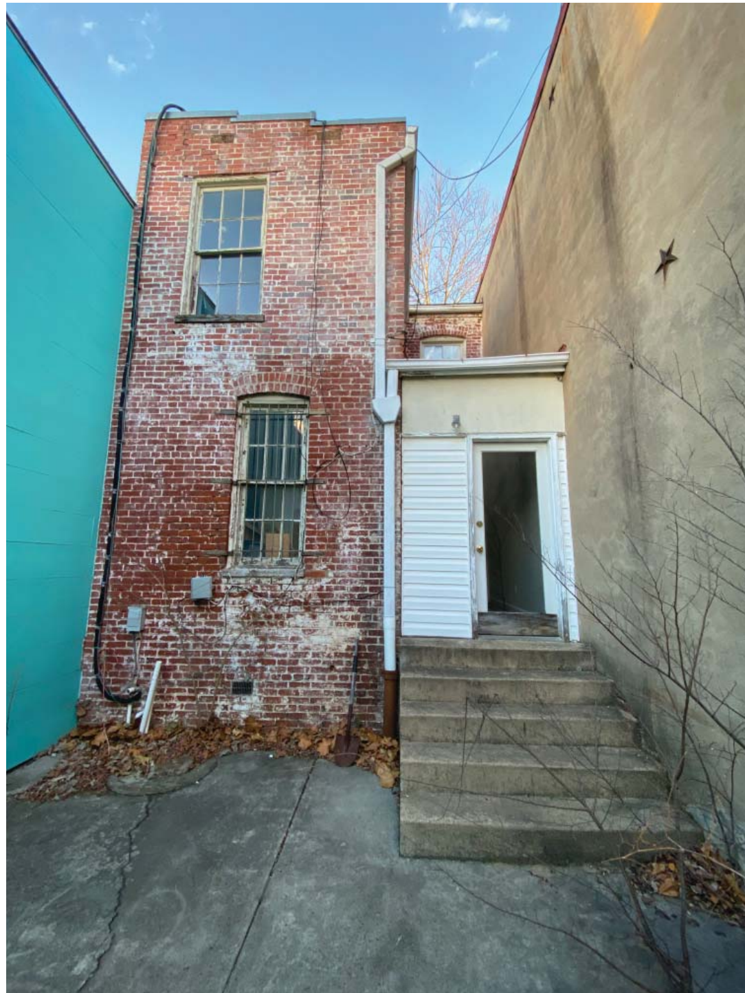
rear facade, close-up
