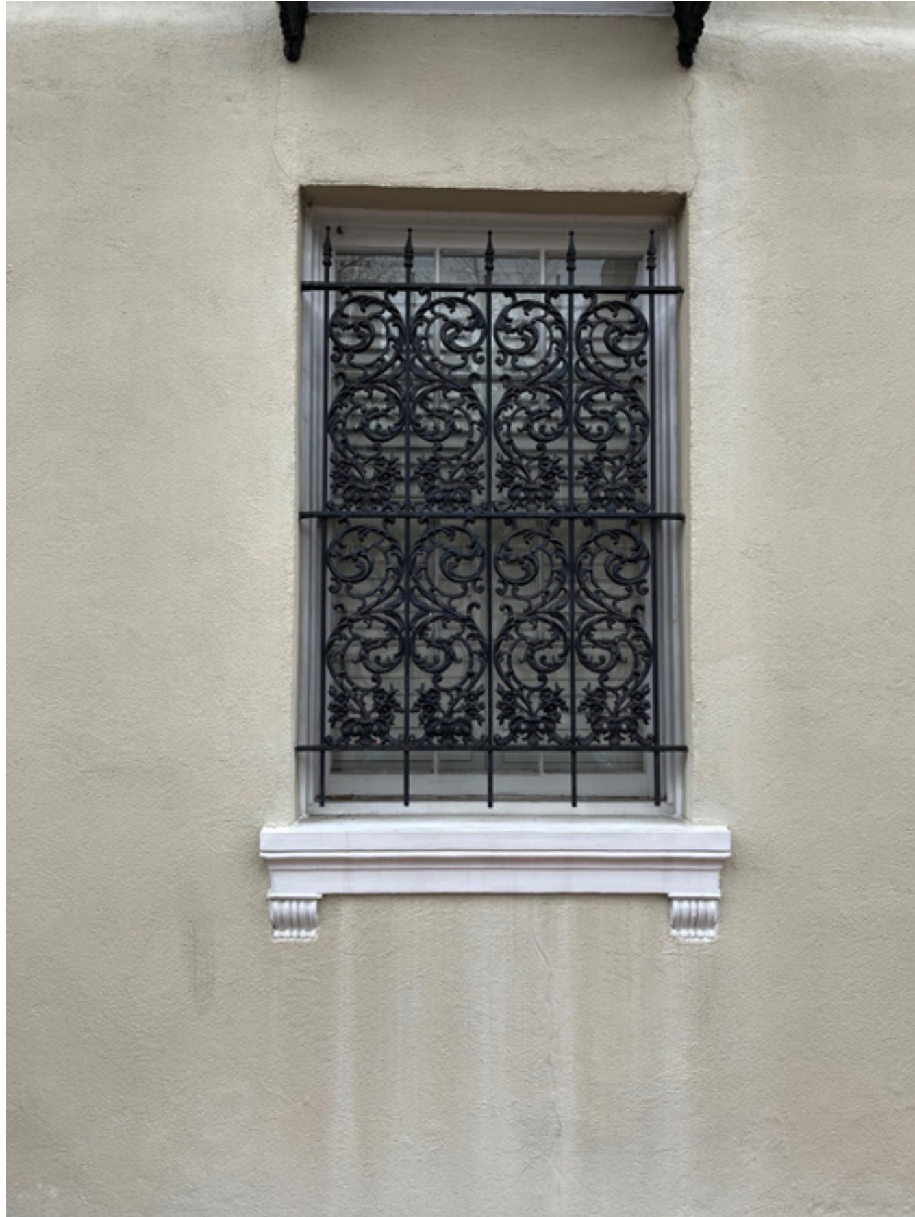
EXISTING FIRST FLOOR WINDOW
