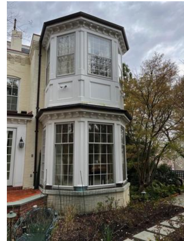
VIEW FROM REAR YARD - EXISTING BAY
