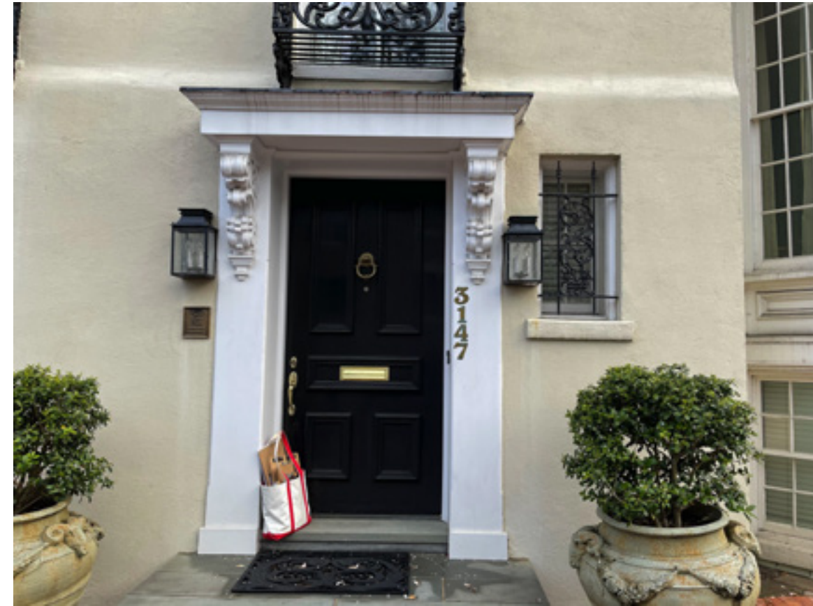
EXISTING FRONT DOOR
