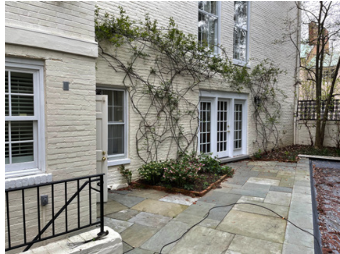
EXISTING SIDE WINDOWS
