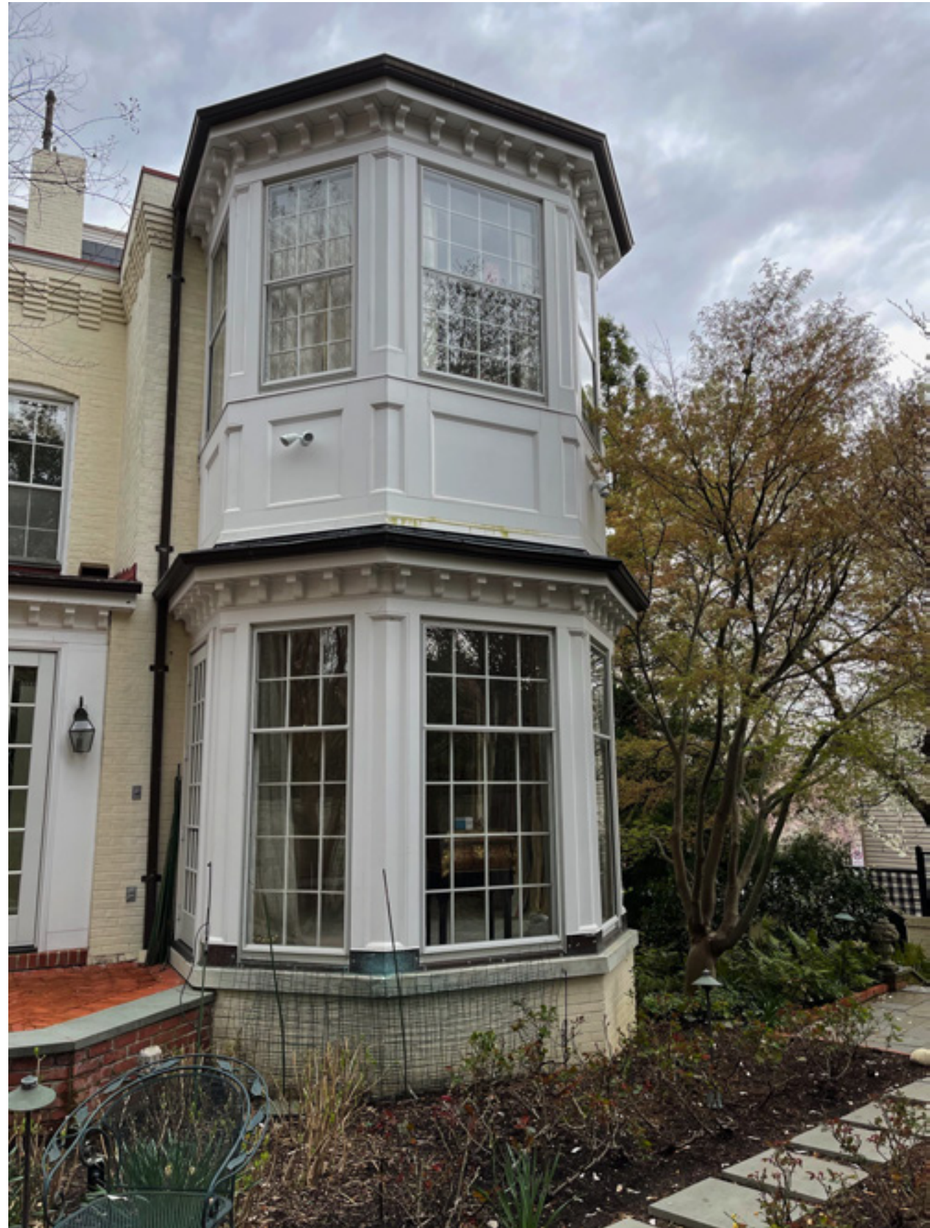
VIEW FROM REAR YARD - EXISTING BAY
