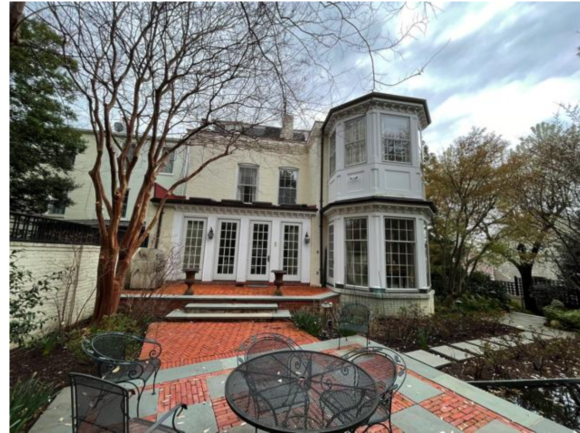
VIEW FROM REAR YARD - OVERALL
