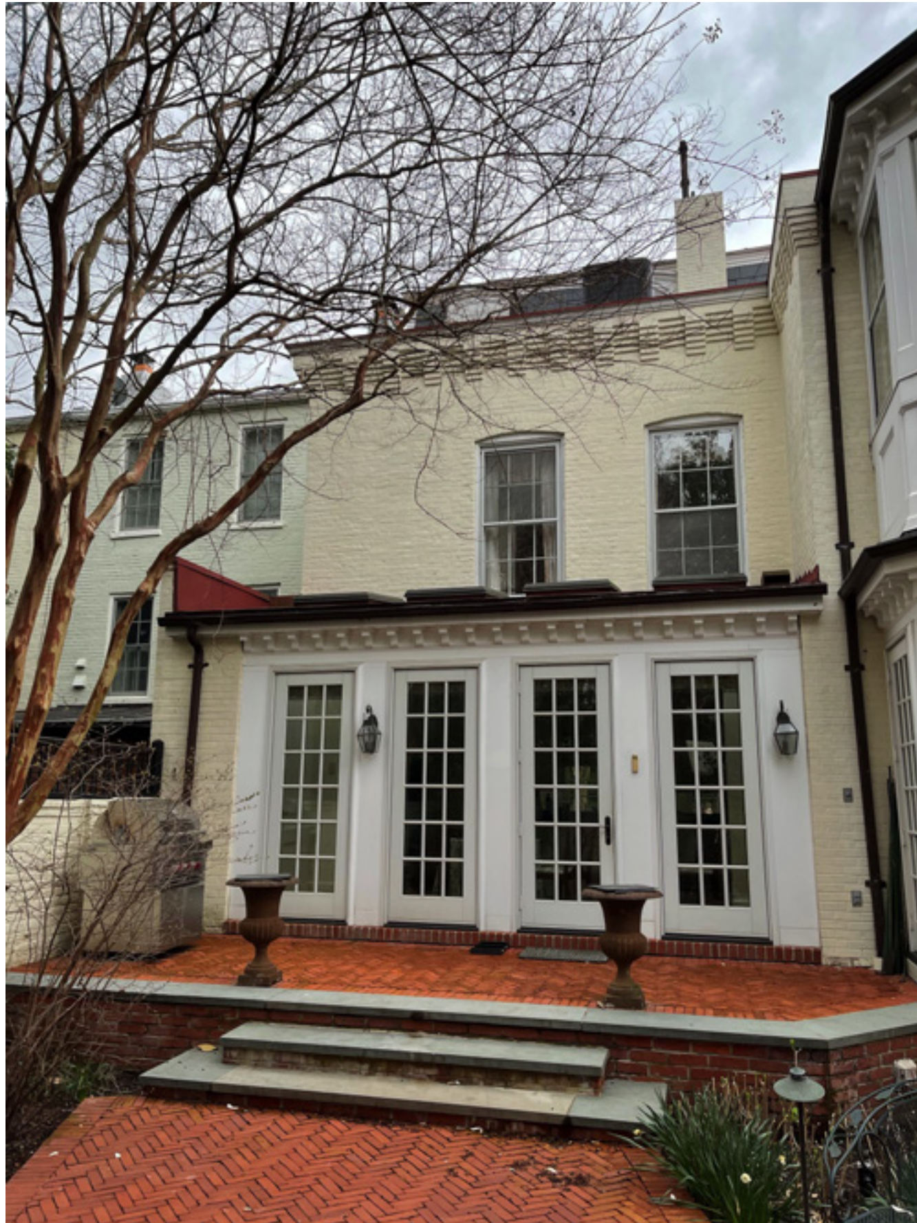
VIEW FROM REAR YARD - EXISTING BREAKFAST ROOM
