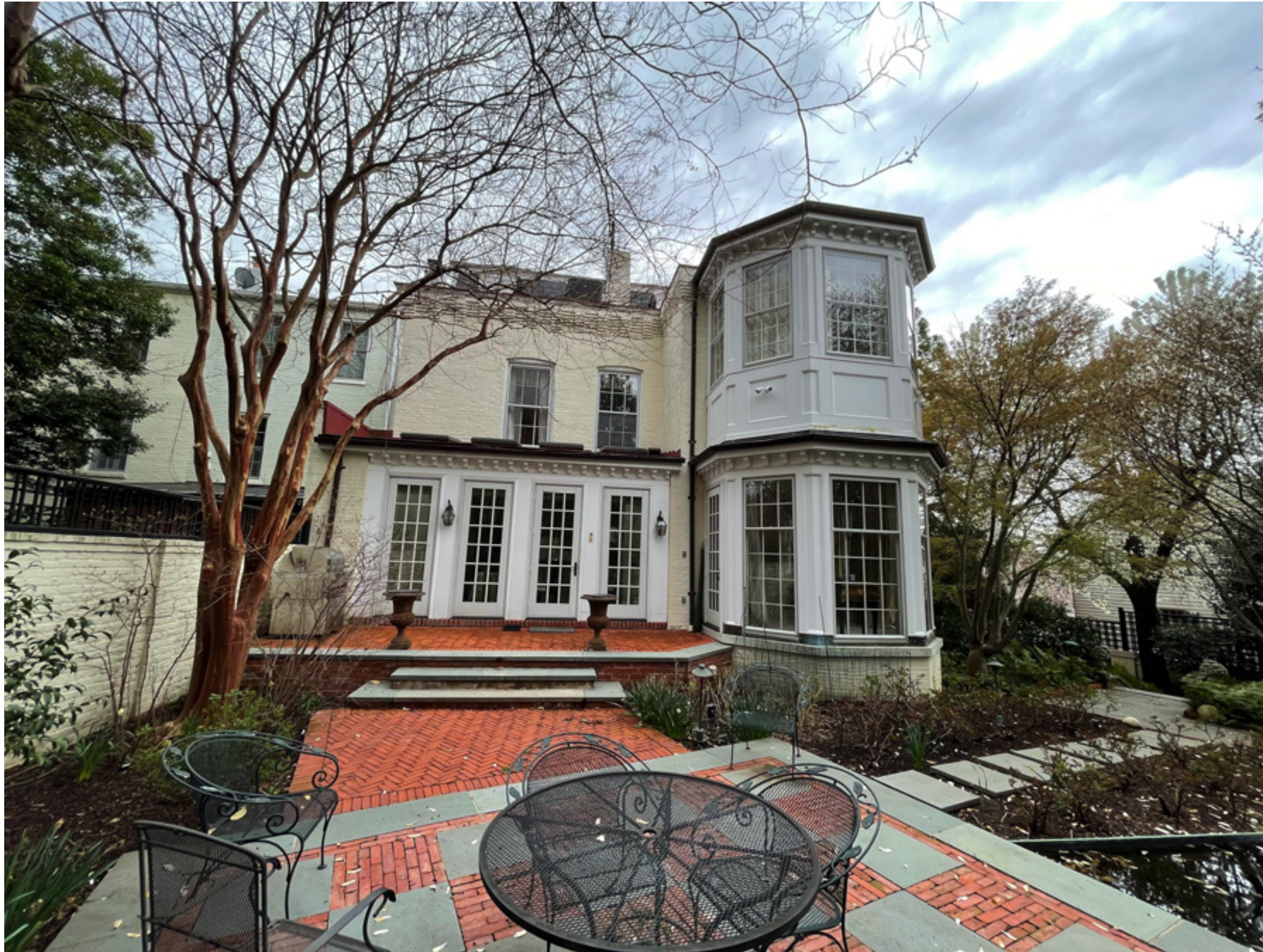
VIEW FROM REAR YARD - OVERALL
