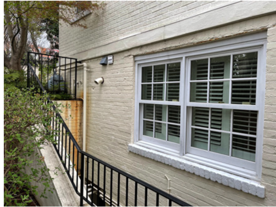
EXISTING WINDOW AT ADDITION
