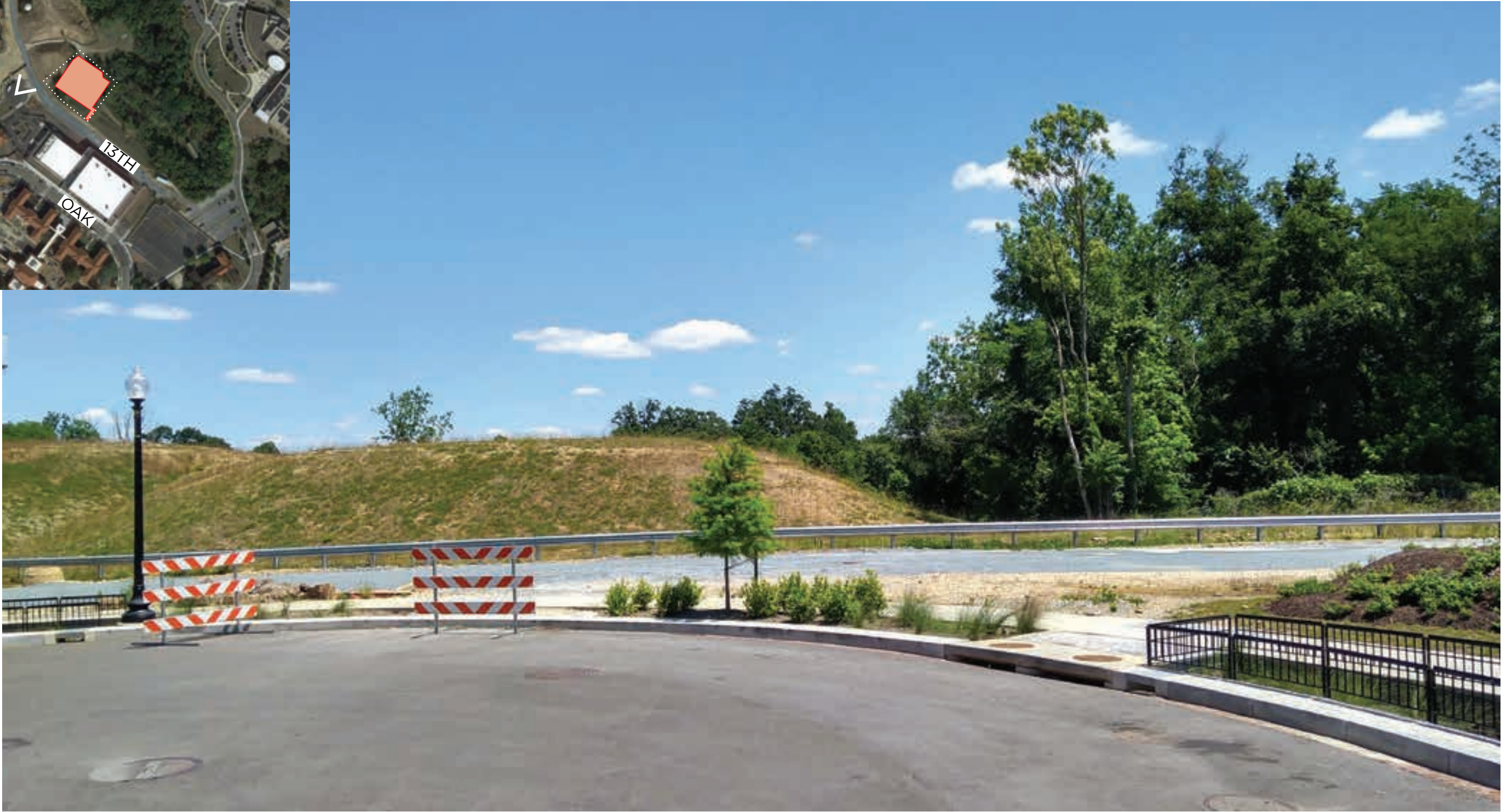
Southwest corner of Site from Cypress Street
