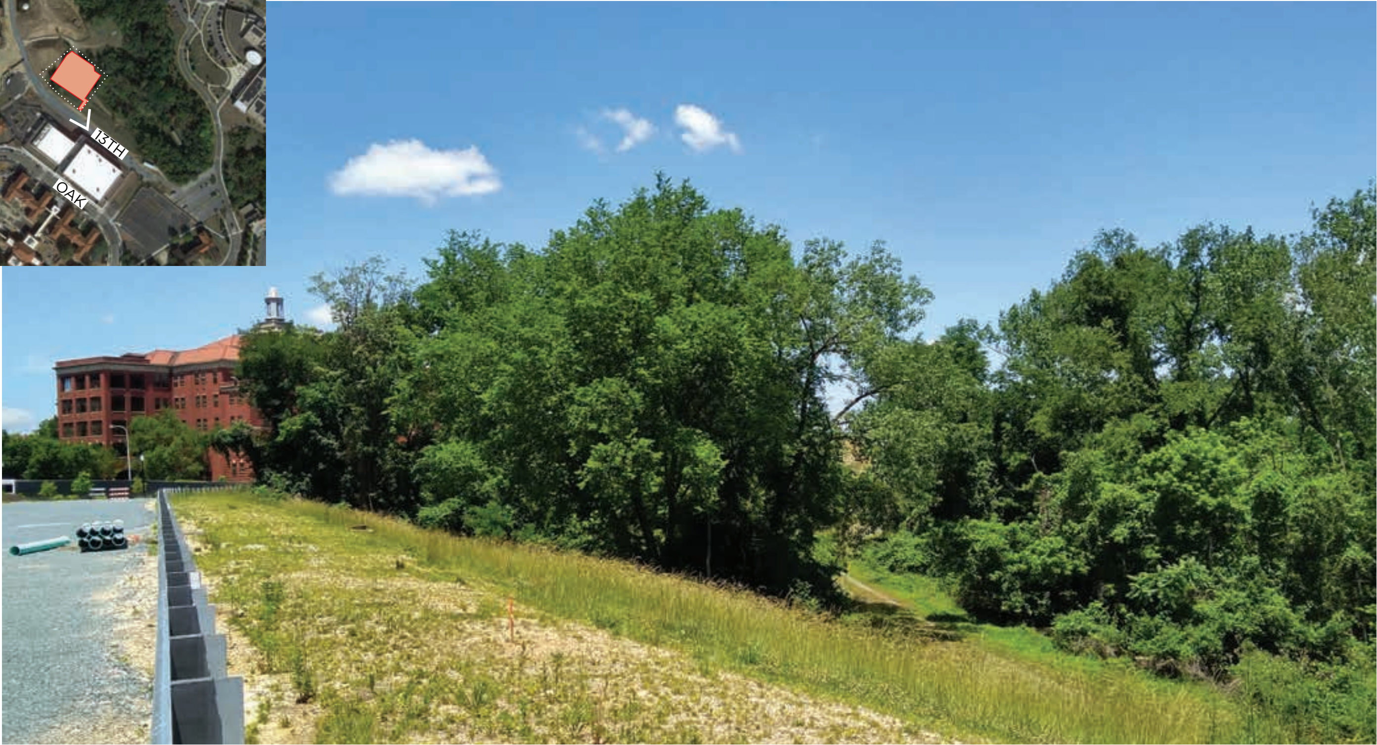
Southeast corner of Site from Temporary 13th Street
