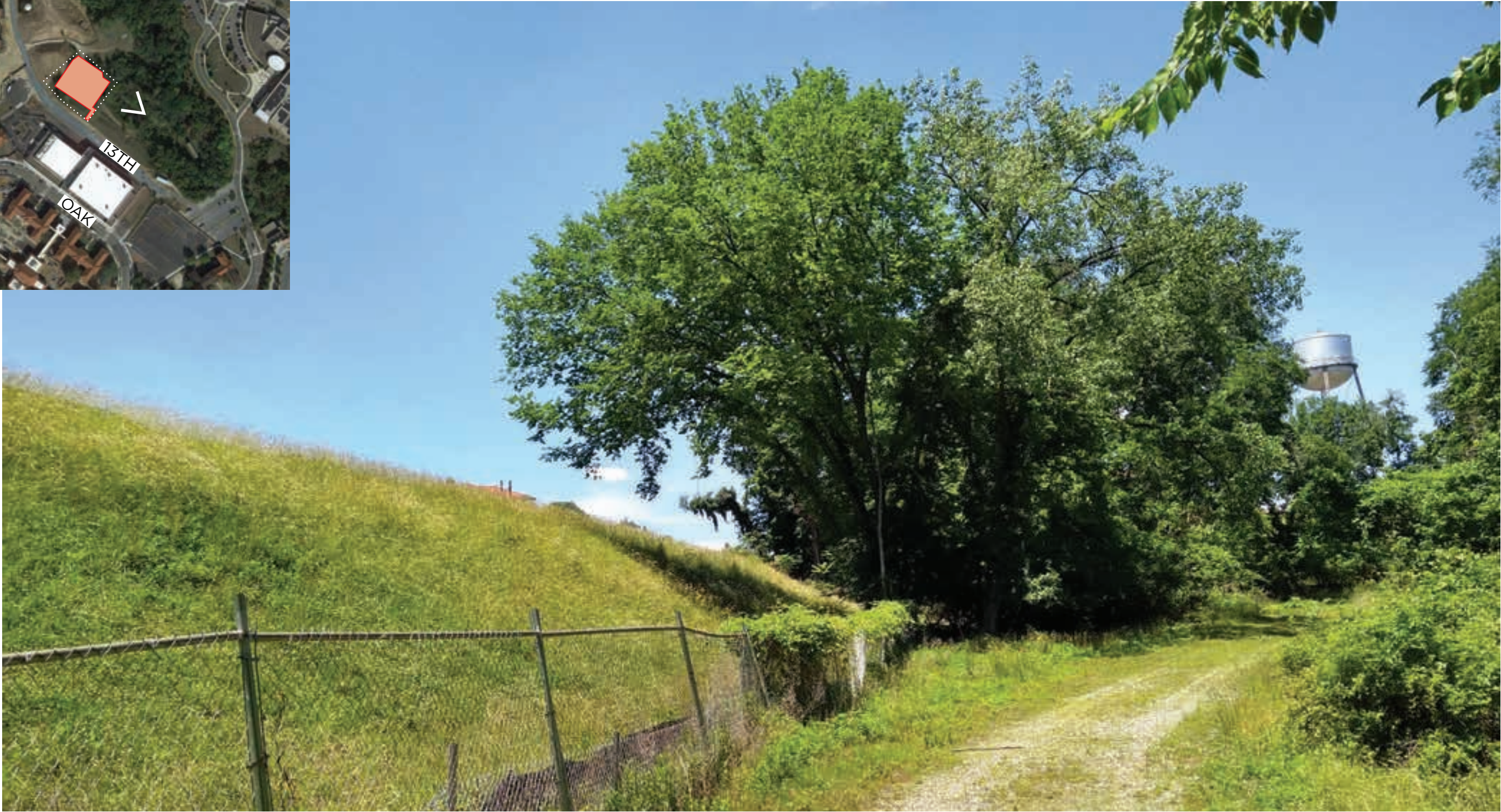
1. Northeast corner of Site from WMATA Access Road
