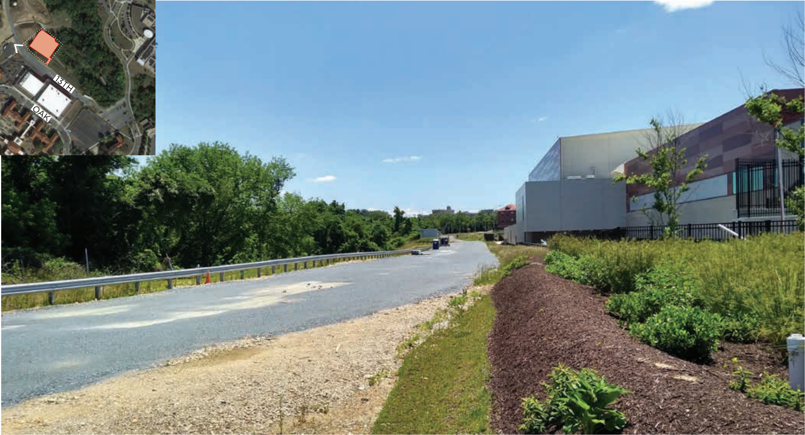
4. Site from Cypress St. & Temp. 13th Street
