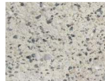
Sandblasted finish at cast-in-place concrete walls
