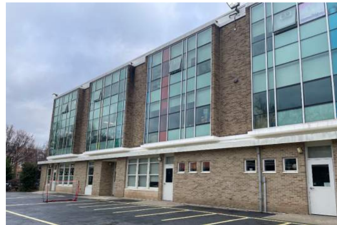
A 3RD ST SE FACADE
