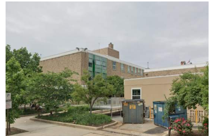
F ENTRANCE AT D ST SE
