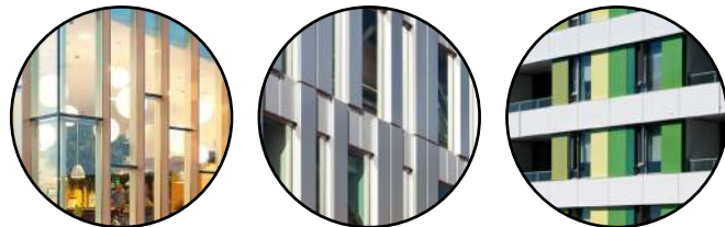
METAL RAINSCREEN PANELS ALUMINUM COMPOSITE MATERIAL (ACM)
