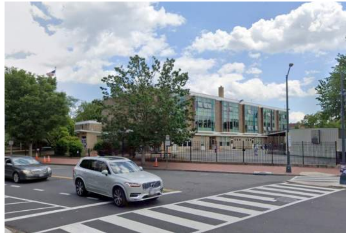
C INTERSECTION AT 3RD ST SE & N CAROLINA AVE SE
