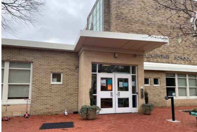
B N CAROLINA AVE SE ENTRANCE
