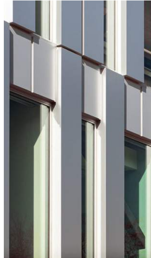
Aluminum Composite Material panels will differentiate the corner material and be expressed in long vertical lines.
