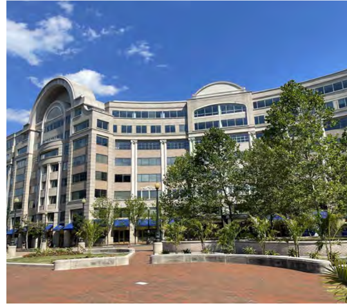
7. MARYLAND AVE FACADE AT CIRCLE
