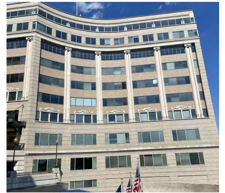
5. SW CORNER AT MAINE AVE
