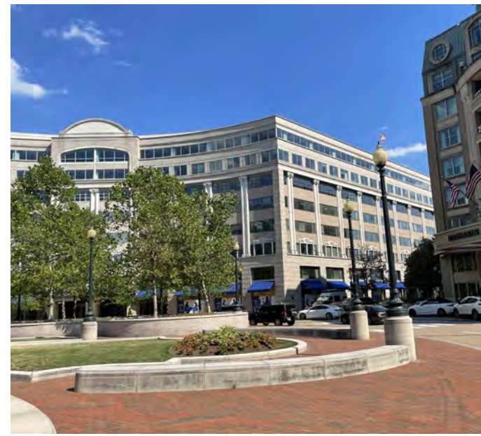
6. MARYLAND AVE FACADE NW CORNER
