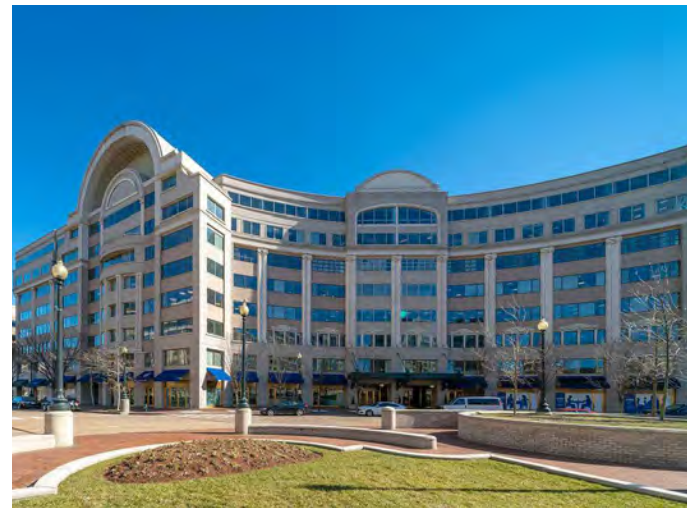
2. MARYLAND AVE FACADE AT CIRCLE
