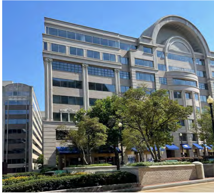
8. MARYLAND AVE FACADE NE CORNER
