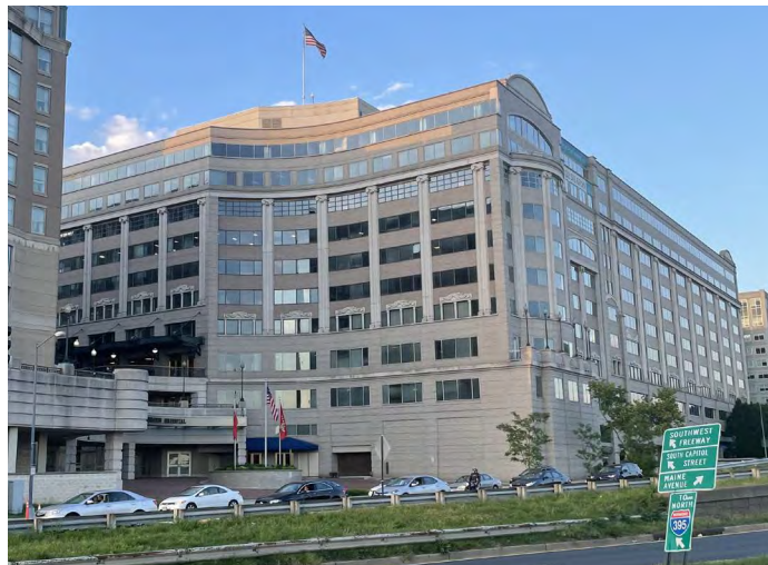
4. WEST FACADE AT SOUTH END
