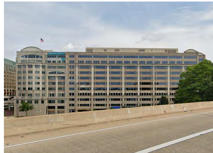
3. SOUTH FACADE FROM 395
