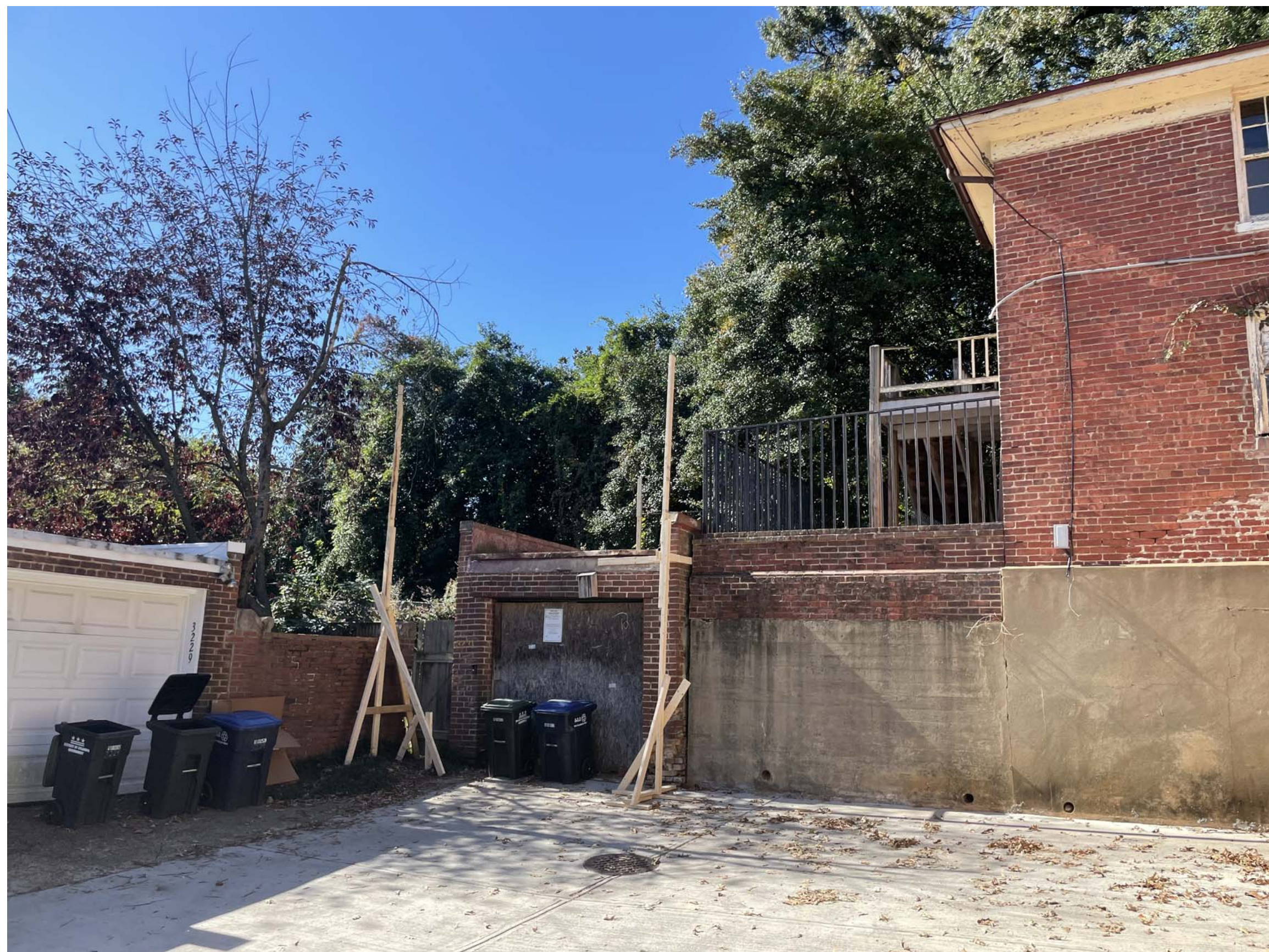
VIEW SOUTHWEST FROM ALLEY
