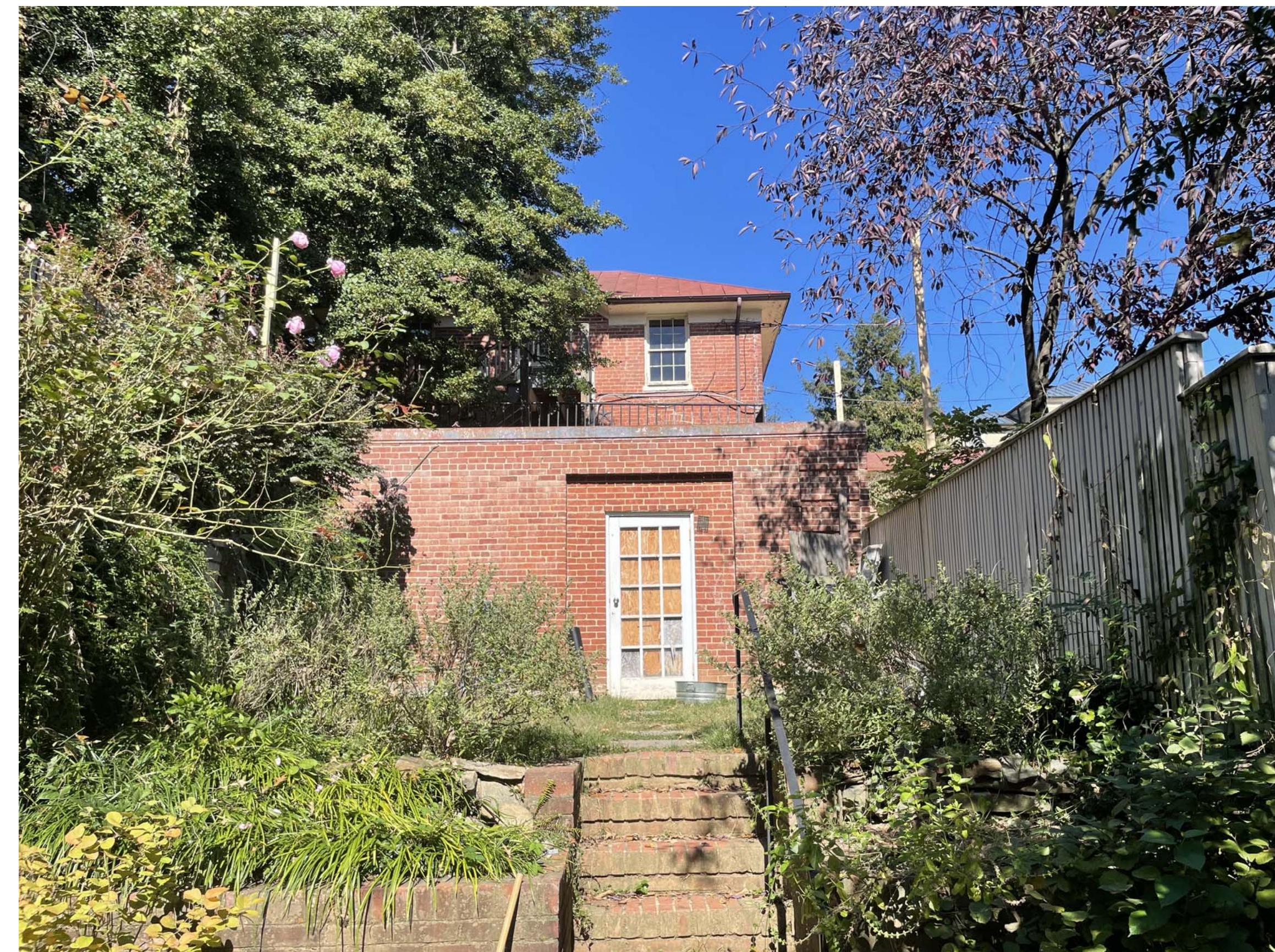
VIEW FROM REAR YARD
