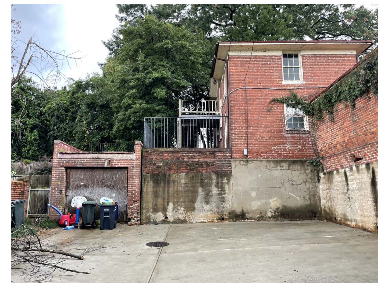
2 - VIEW OF CARRIAGE HOUSE TO THE NORTH
