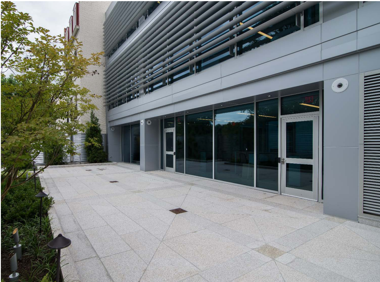
REAR TERRACE- EXISTING 2406 MASSACHUSETTS AVENUE
