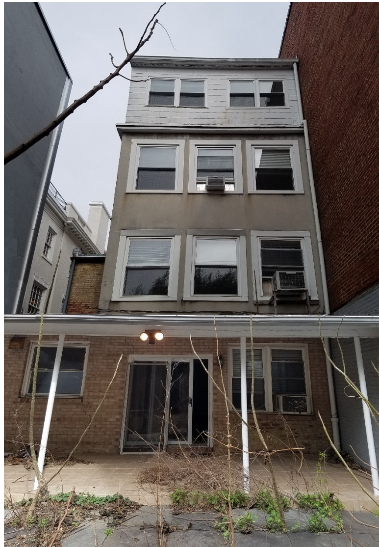
REAR TERRACE- EXISTING 2400 MASSACHUSETTS AVENUE
