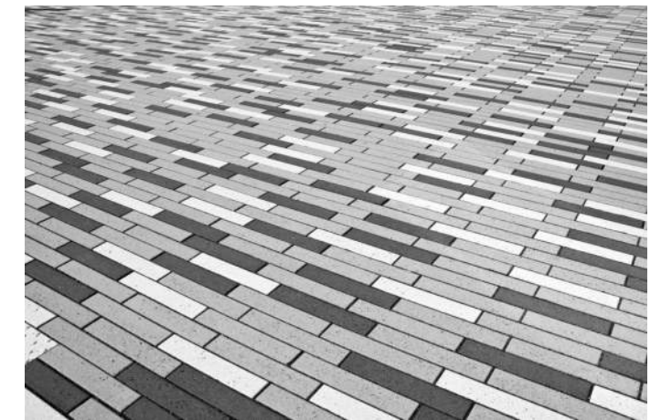
Unit Pavers Location: Entry Plaza, Playground Plaza, Outdoor Courtyards
