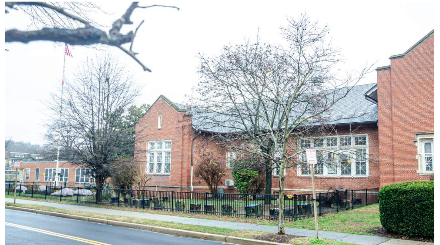
2 MONROE ST LOOKING WEST
