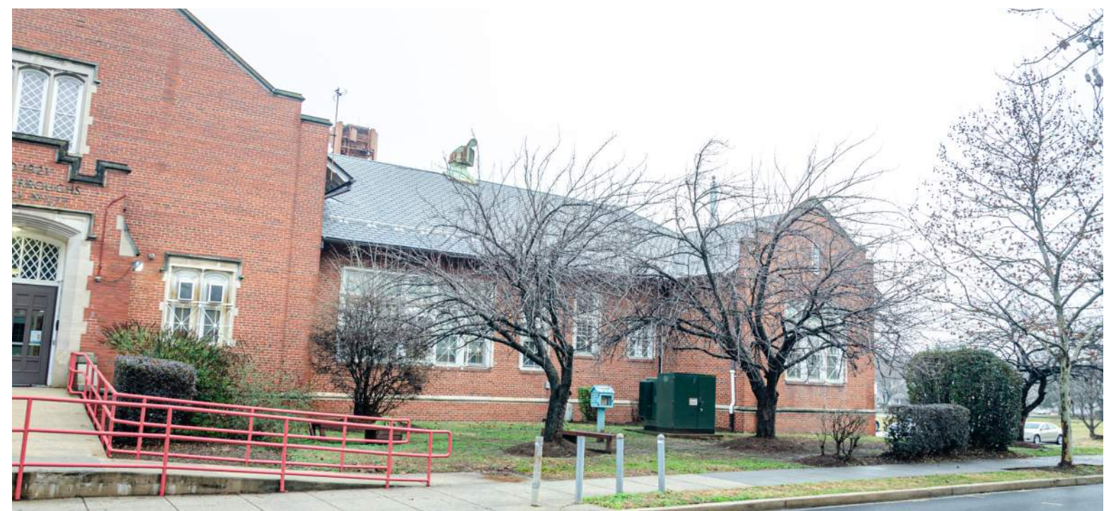
4 MONROE ENTRANCE LOOKING EAST
