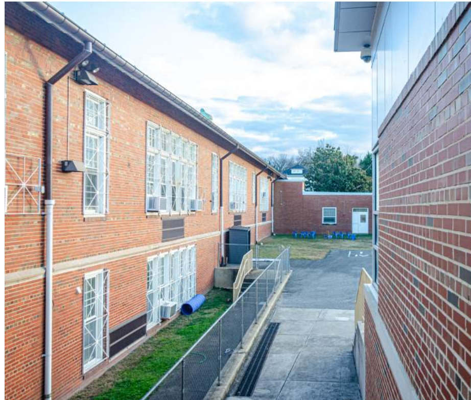
1 WEST HISTORIC FACADE
