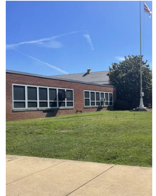
3 SOUTH FACADE OF 1959 ADDITION.
