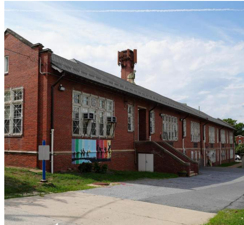
2 SOUTH EAST FACADE FROM MONROE ST
