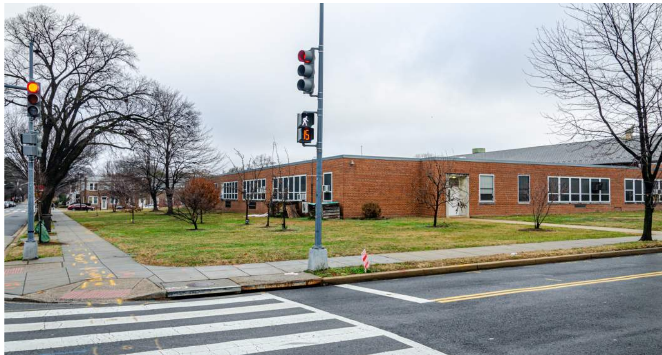
4 CORNER OF MONROE ST AND 18H ST NE, LOOKING AT 1959 ADDITION.
