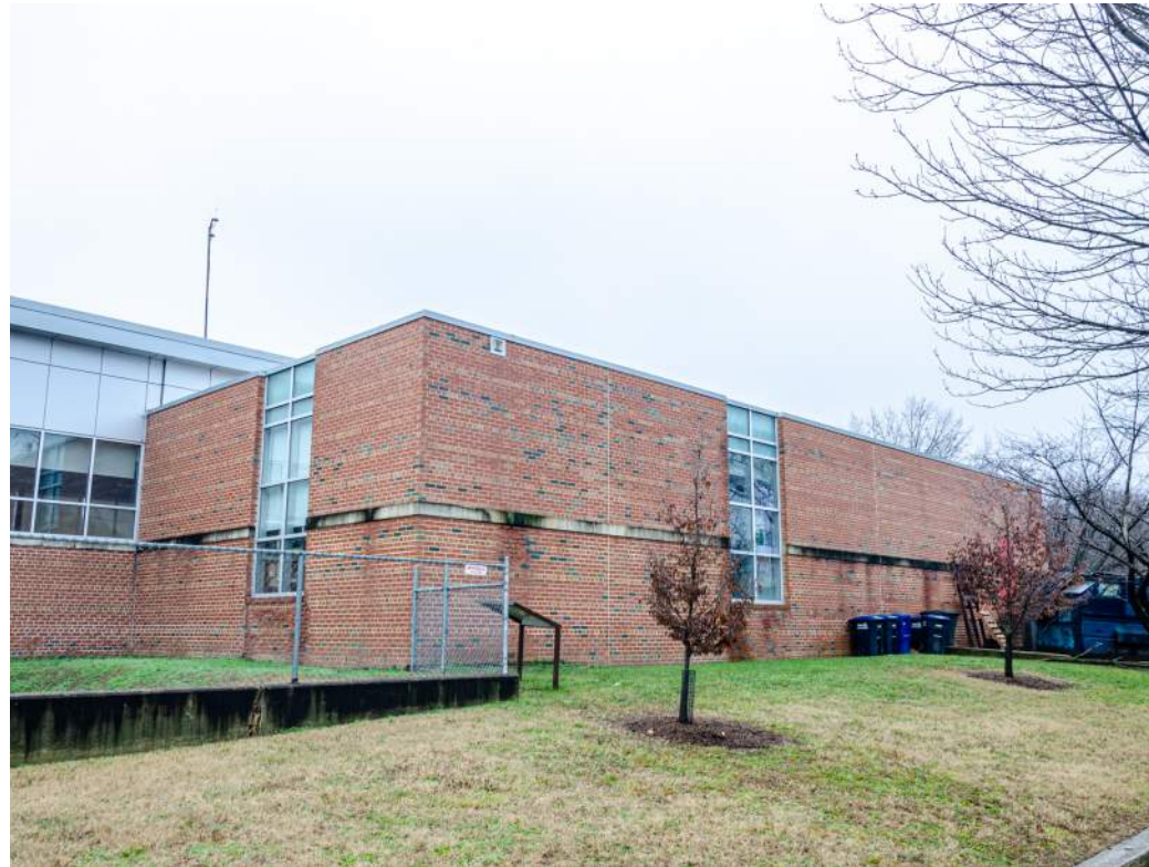
1 NORTH FACADE OF 2013 ADDITION.
