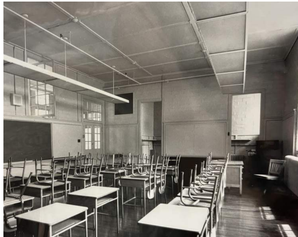
Historic photo of classroom showing corridor ventilation window (top left).
