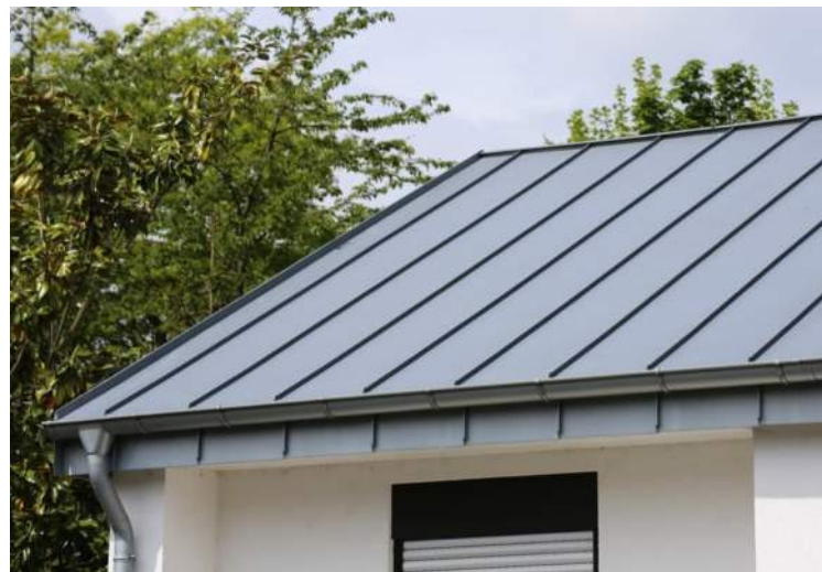
Standing Seam Metal Roof Location: Addition
