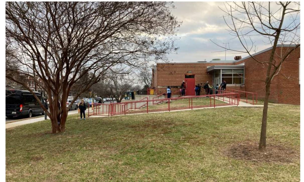
5 RAMP AND NEWTON ST ENTRANCE OF 2013 ADDITION.
