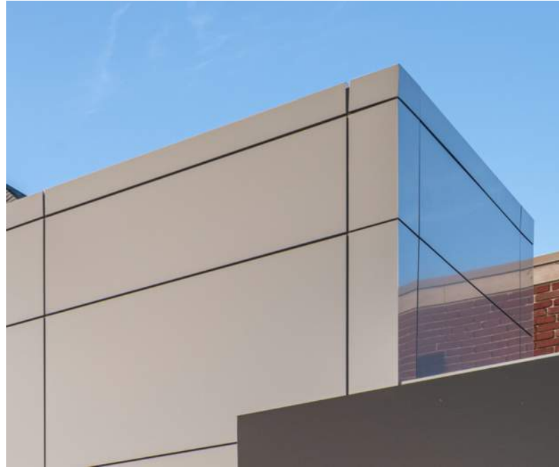
Prefinished Alum Metal Panel Location: Addition
