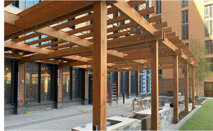
Shade Structure over Grilling Area
